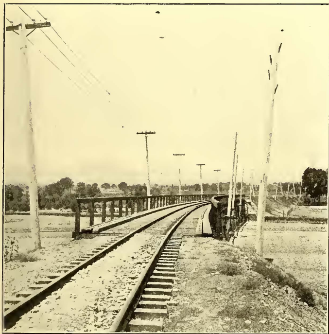
FIG. 8.—400-FT. BRIDGE ACROSS CLEAR CREEK
