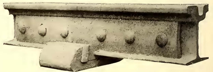
FIG. 2.—RAIL-JOINT ATTACHED TO RAIL
