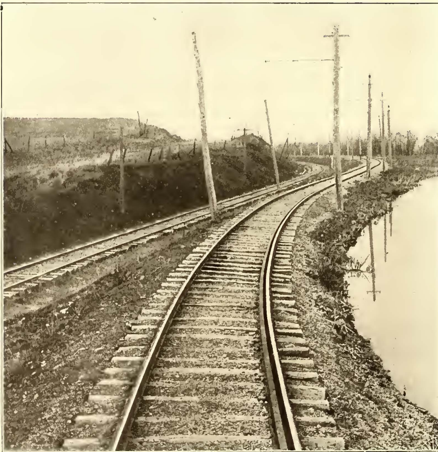
REVERSE CURVE ON C., B. L. & N. RAILWAY, WHERE IT PASSES CANAL ON ONE SIDE AND THE STEAM LINE AND HIGHWAY ON THE OTHER
