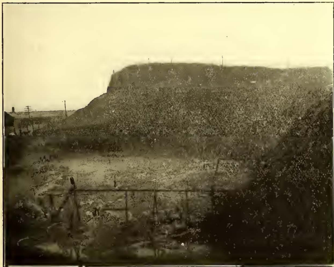
FIG. 3.—POWER-HOUSE SITE ON NOV. 15, 1902
