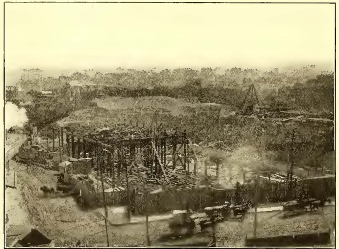
FIG. 4.—POWER-HOUSE STRUCTURE ON MARCH 25, 1903
