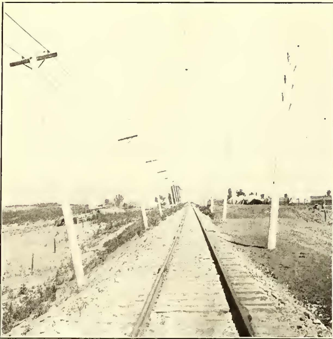
FIG. 5.—VIEW SHOWING TRACK AND OVERHEAD CONSTRUCTION
