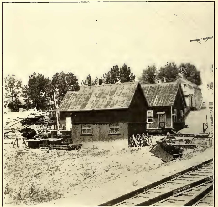
FIG. 6.—STORAGE YARD, FREIGHT HOUSE AND DISPATCHER'S OFFICE AT ARVADA
