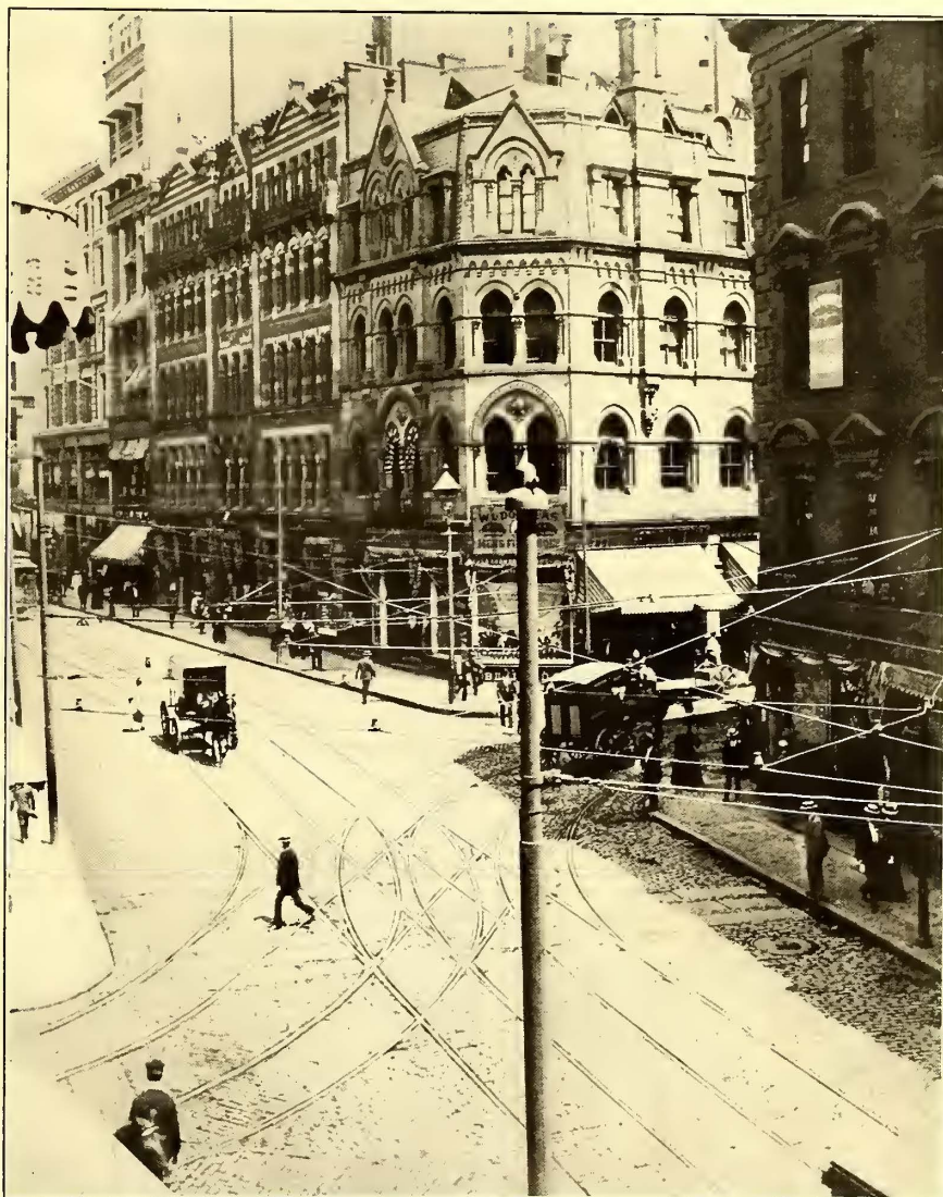
COMPLICATED TRACK AND SPECIAL WORK CONSTRUCTION IN NARROW STREETS IN BOSTON
