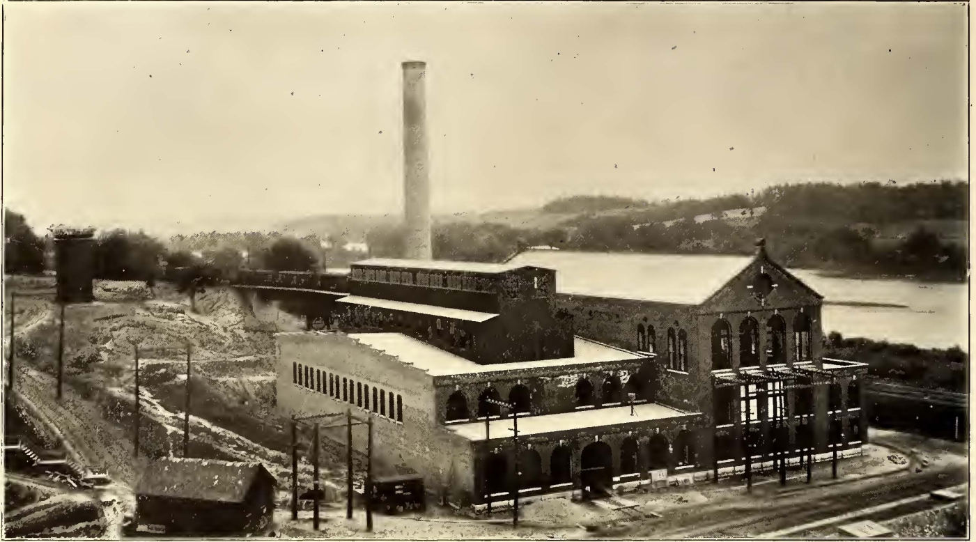
MAIN POWER HOUSE AT TRIBE'S HILL
