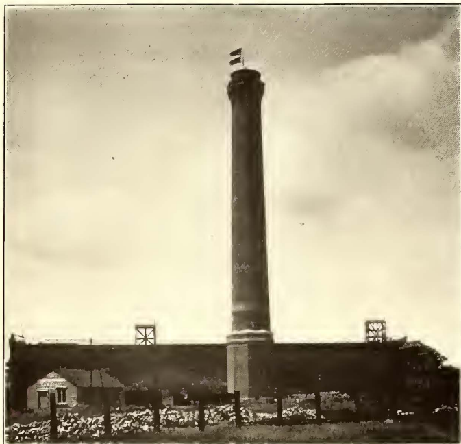
METROPOLITAN POWER HOUSE, WITH AMERICAN AND ENGLISH FLAGS ABOVE STACK
