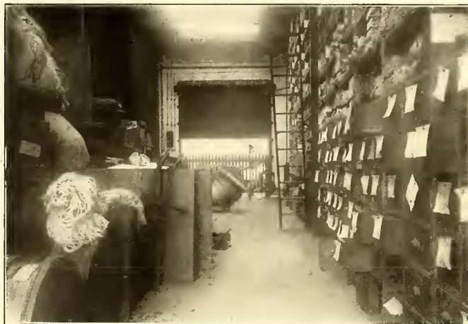
STOCK ROOM AT NORTH ALBANY SHOP
