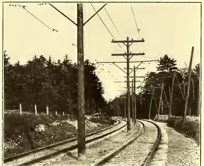
LINE VIEW NEAR JOHNSTOWN, SHOWING TRACK AND OVERHEAD CONSTRUCTION
