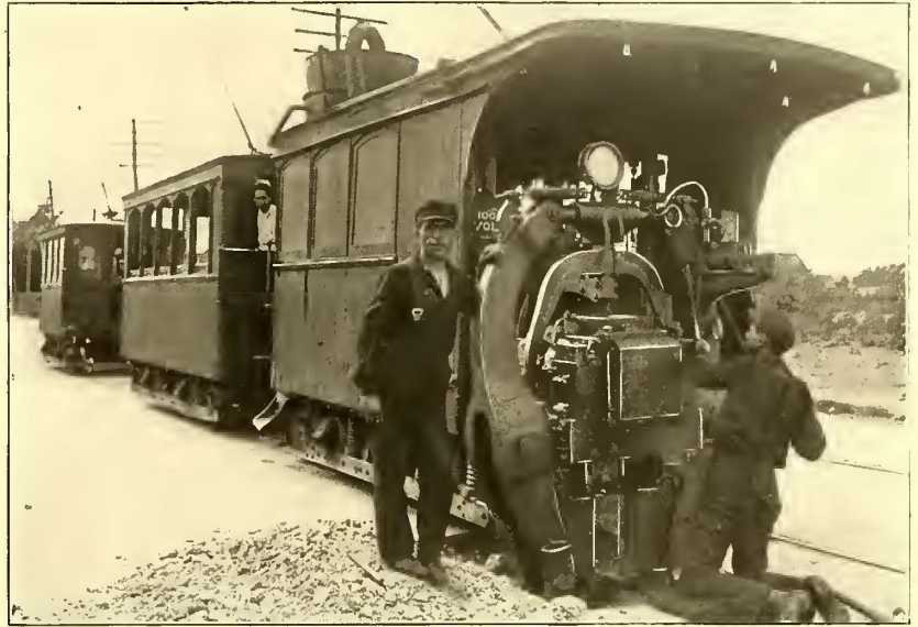
ELECTRICALLY WELDING RAIL JOINTS IN BUFFALO
