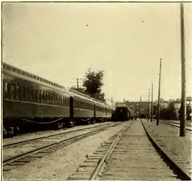
STEAM AND ELECTRIC LINES ENTERING GLOVERSVILLE ON SAME RIGHT OF WAY
