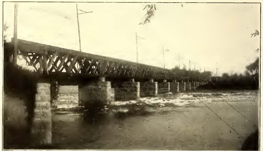
STEEL BRIDGE CROSSING HUDSON RIVER
