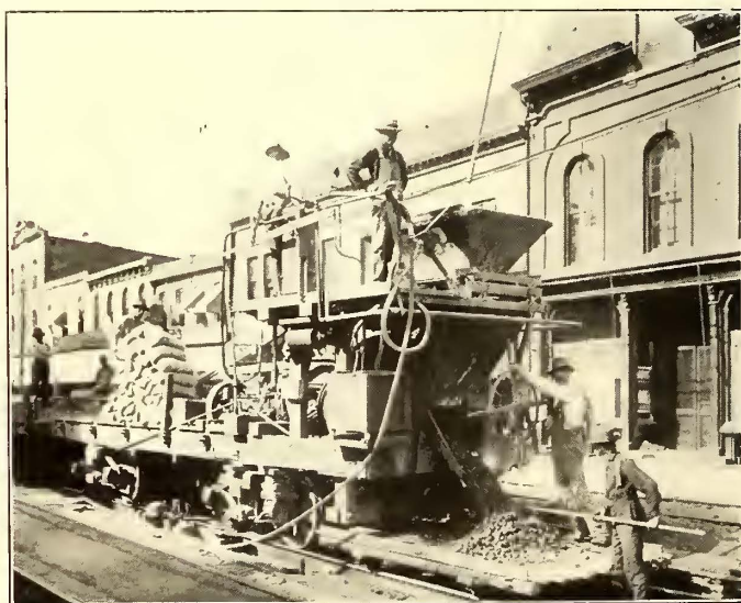
CONCRETE MIXER USED IN TRACK CONSTRUCTION IN DETROIT
