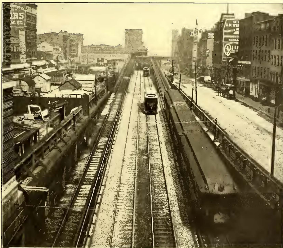
INCLINE AT NORTH STATION, BOSTON, SHOWING CONNECTION BETWEEN SUBWAY, SURFACE AND ELEVATED TRACKS
