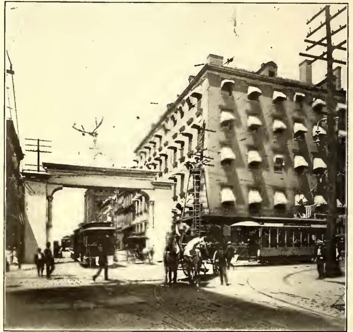
CORNER EUTAW AND BALTIMORE STREETS, SHOWING OVERHEAD CONSTRUCTION
