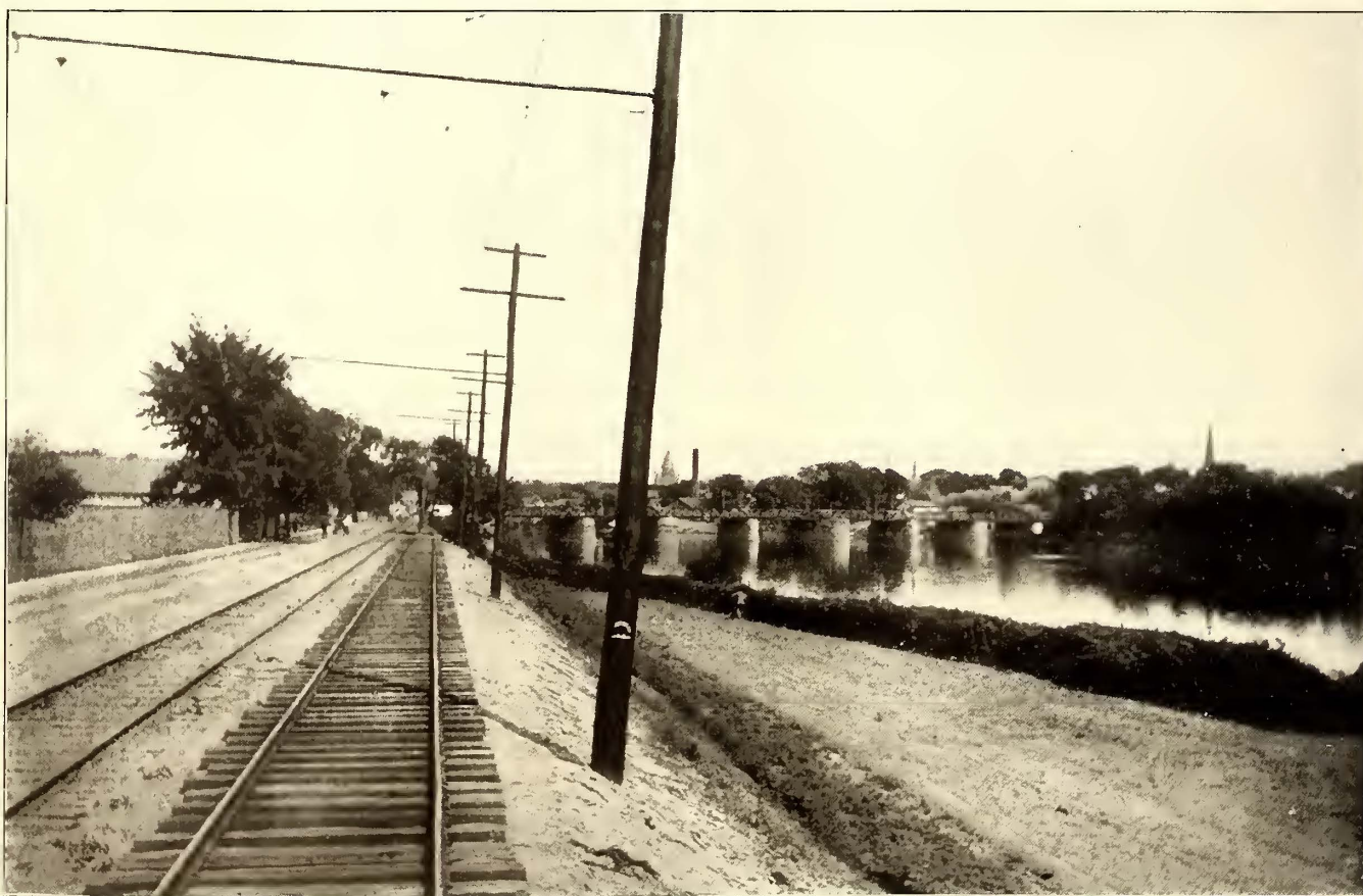
LINE CONSTRUCTION FOR DOUBLE-TRACK, WITH POLE AT ONE SIDE—BRIDGE CROSSING MOHAWK RIVER
