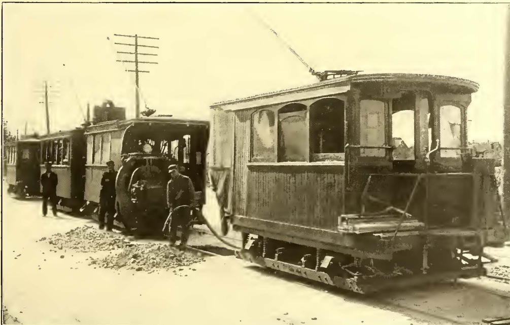
SAND BLAST CAR AND ELECTRIC TRACK JOINT WELDING APPARATUS IN BUFFALO
