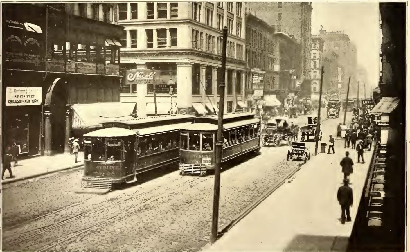
VIEW ON CLARK STREET, NEAR ADAMS, CHICAGO, SHOWING STANDARD OVERHEAD CONSTRUCTION IN DOWN-STREETS
