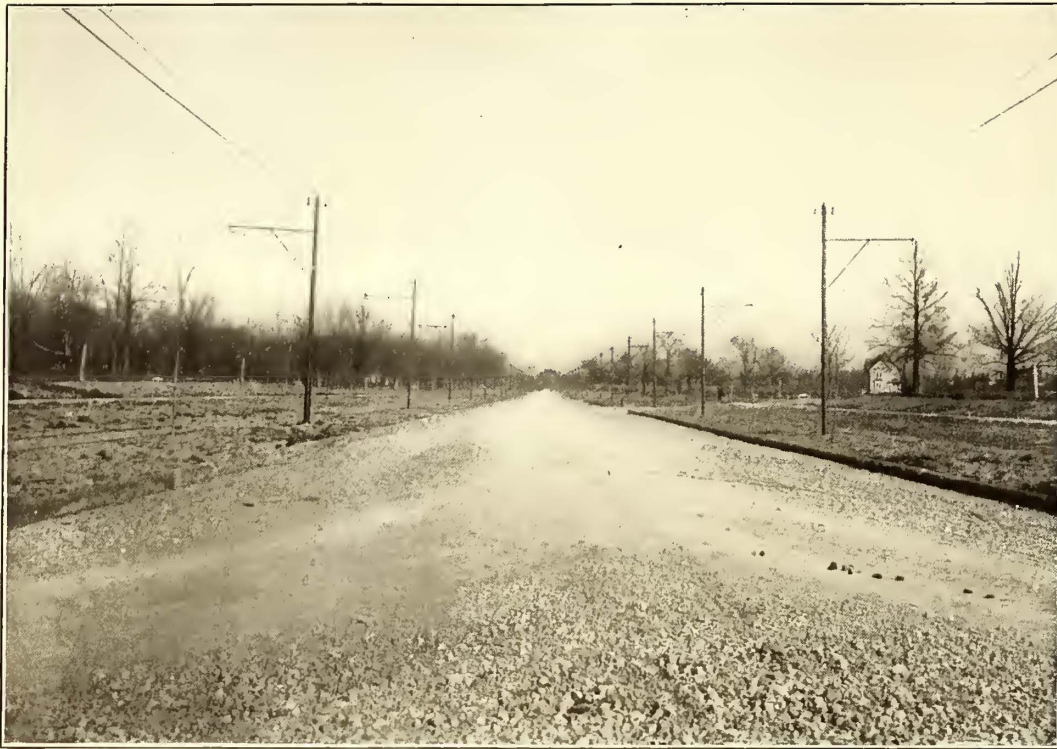
VIEW OF CLIFTON BOULEVARD, CLEVELAND, SHOWING PART OF 5 1/2 MILES OF DOUBLE TRACK ROAD RECENTLY BUILT BY THE CLEVELAND ELECTRIC RAILWAY COMPANY
