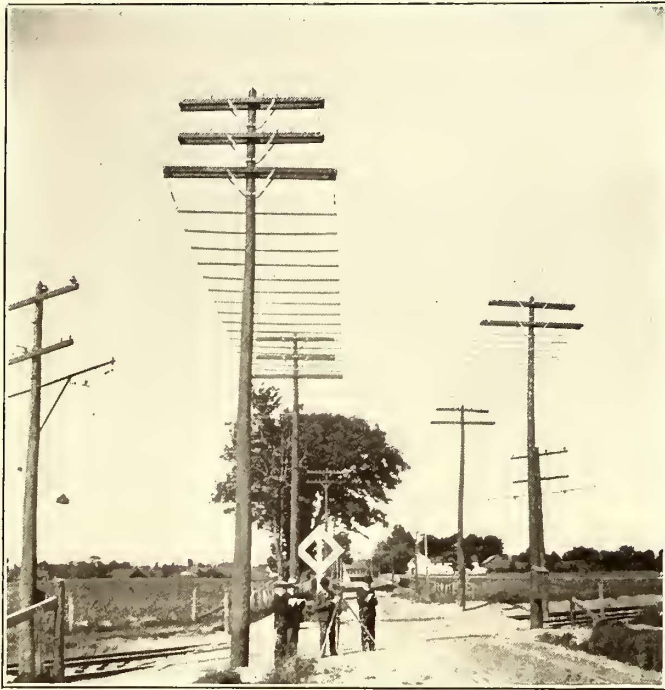
PROTECTING WIRES AT RAILROAD CROSSING
