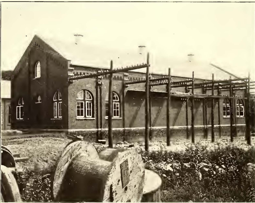
AMSTERDAM SUB-STATION, SHOWING HIGH-TENSION LINE SUPPORTS
