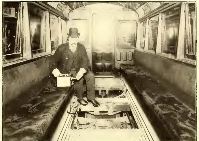
FIG. 2.—USING MOTOR TESTER ON CAR
