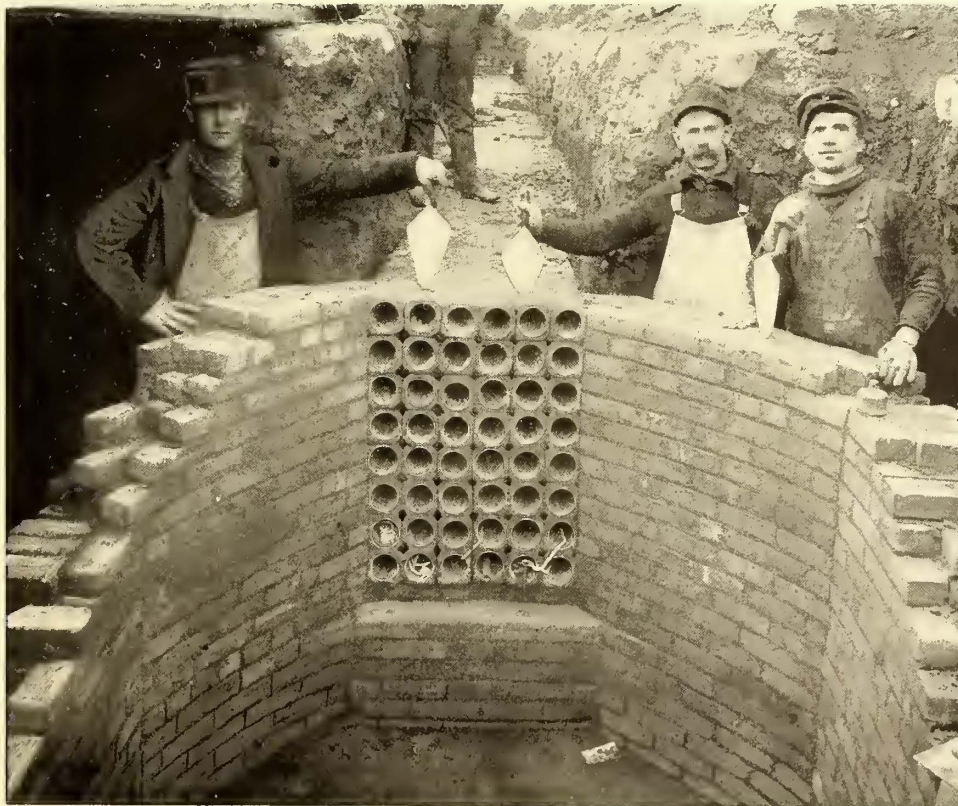
LAYING CONDUIT IN BROOKLYN
