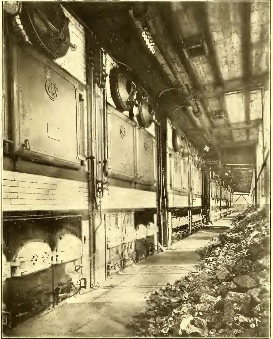
BOILER ROOM, SHOWING SETTINGS AND COAL BUNKER CONSTRUCTION
