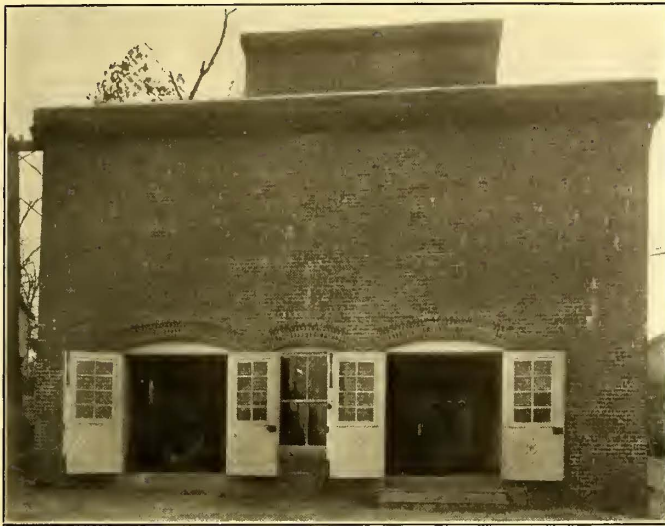
SUB-STATION AT UNIONTOWN.
