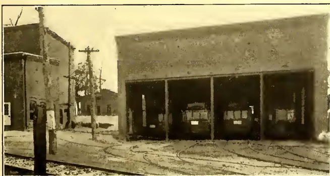
CAR HOUSE, BATTERY HOUSE AND SUB-STATION AT UNIONTOWN
