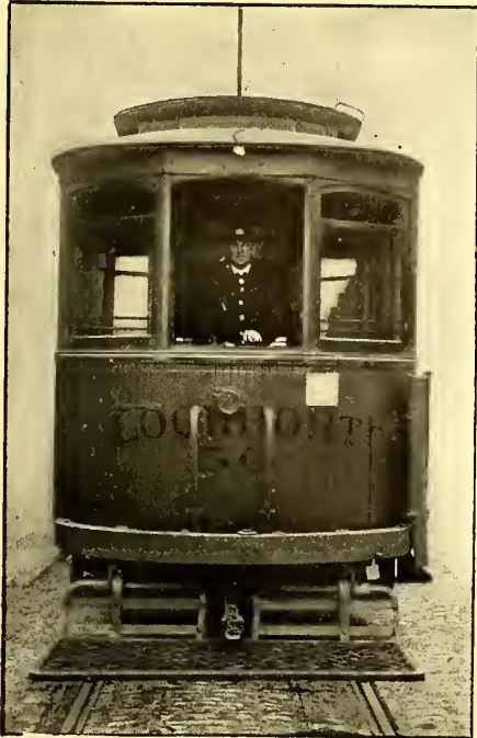
PLATE 13.—FRONT END REGULAR TRAIN, WITH RED DASH SIGN, BY DAY—SEE RULE I-11
