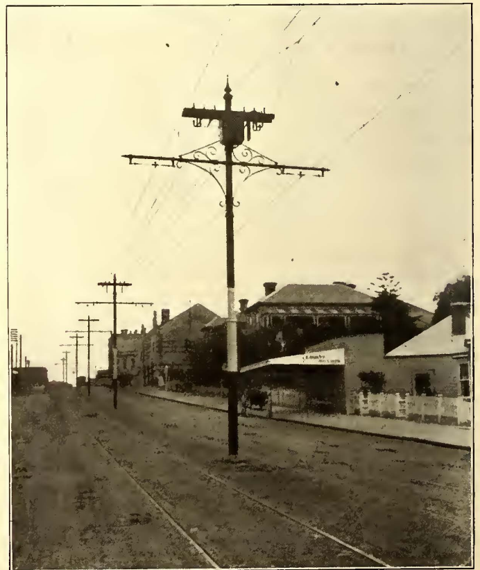
CENTER POLE OVERHEAD CONSTRUCTION
