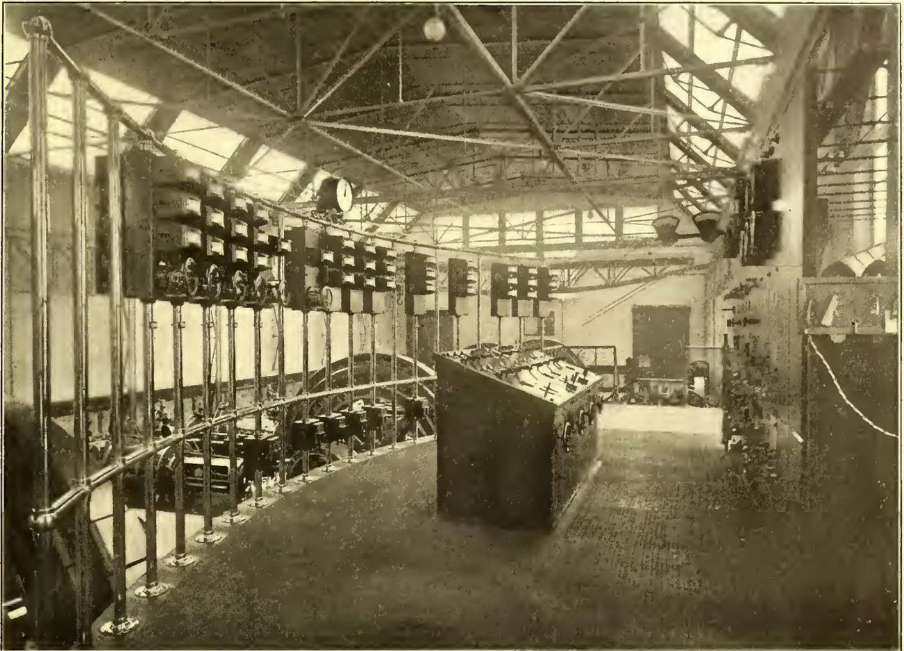
FIG. 5.—SWITCHBOARD GALLERY IN MAIN STATION, WITH DIRECT-CURRENT APPARATUS AT RIGHT, BENCHBOARD IN CENTER, AND ALTERNATING-CURRENT MEASURING INSTRUMENTS ON FRAMEWORK AT LEFT
