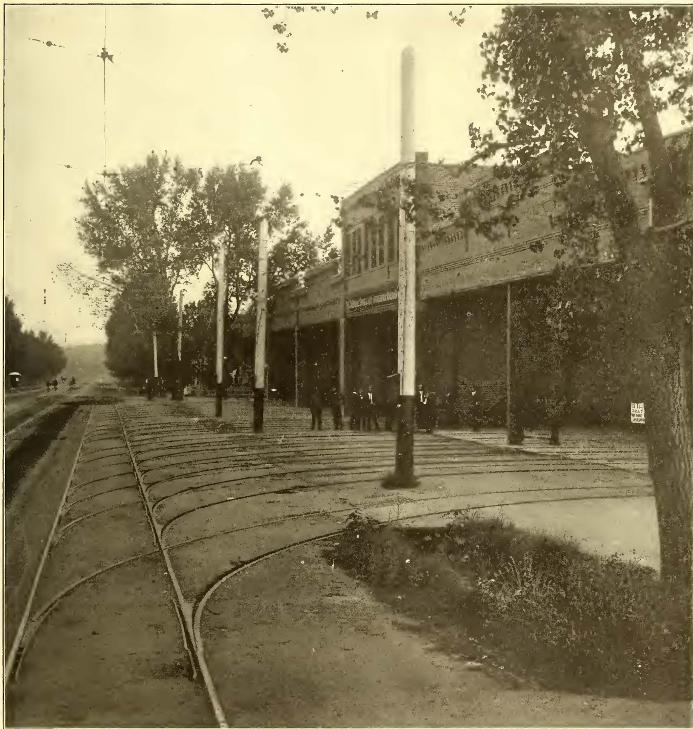
SPECIAL WORK AT CAR HOUSE OF COLORADO SPRINGS & INTERURBAN RAILWAY
