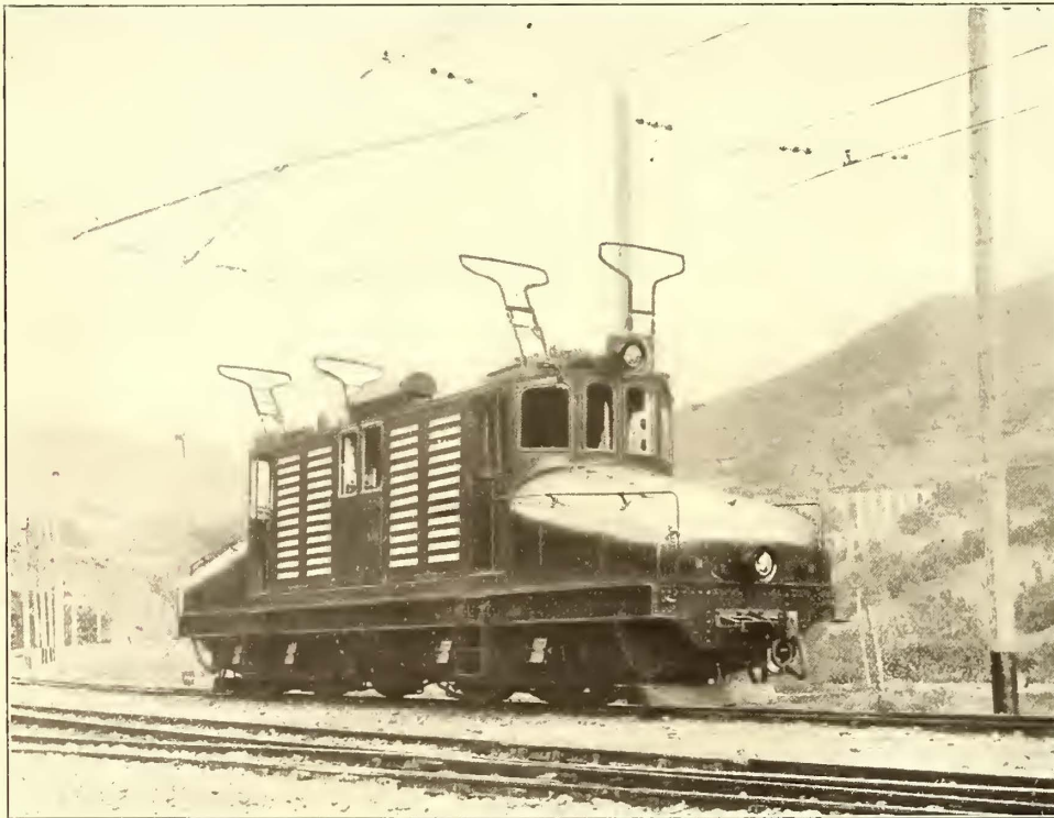
FIG. 2.—OVERHEAD CONSTRUCTION FOR ELECTRIC LOCOMOTIVE
