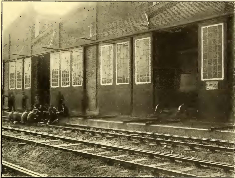
FIG. 16.—TROLLEY WIRE AND CHANNEL-IRON CONDUCTORS AT FRONT OF SHOP
