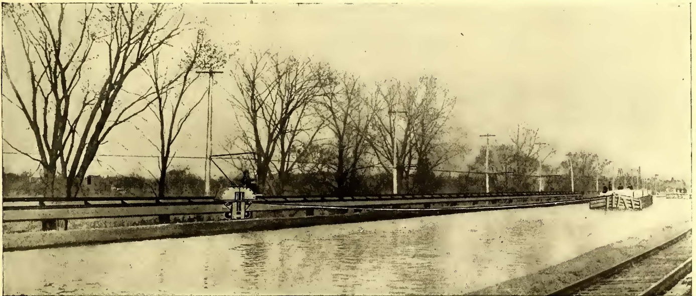
CONSTRUCTION OF TRACK AND POLE LINE
