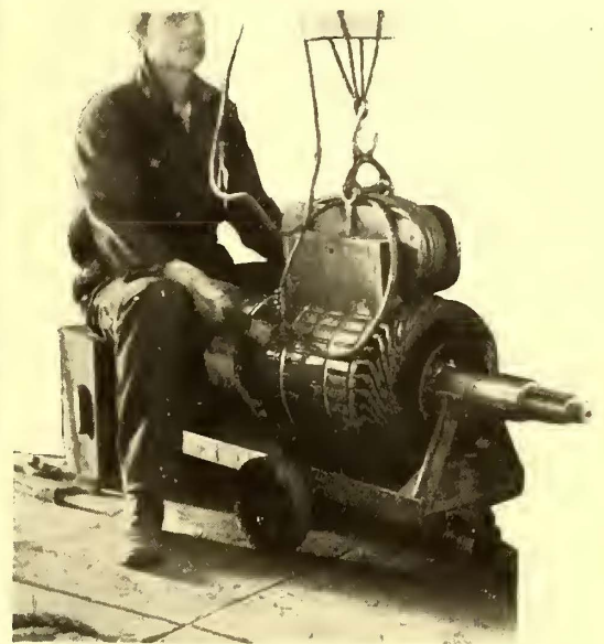
FIG. 20.—TESTING FOR SHORT-CIRCUITED COILS WITH TRANSFORMER
