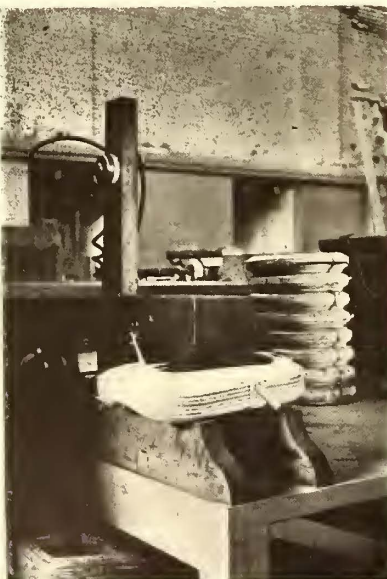
FIG. 21.—TRANSFORMER FOR TESTING FIELD COILS
