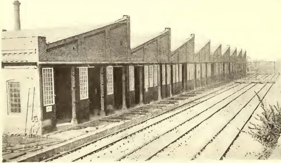
FIG. 1.—GENERAL VIEW OF FRONT OF SHOP AND TRANSFER TABLES, FROM THE SOUTHEAST
