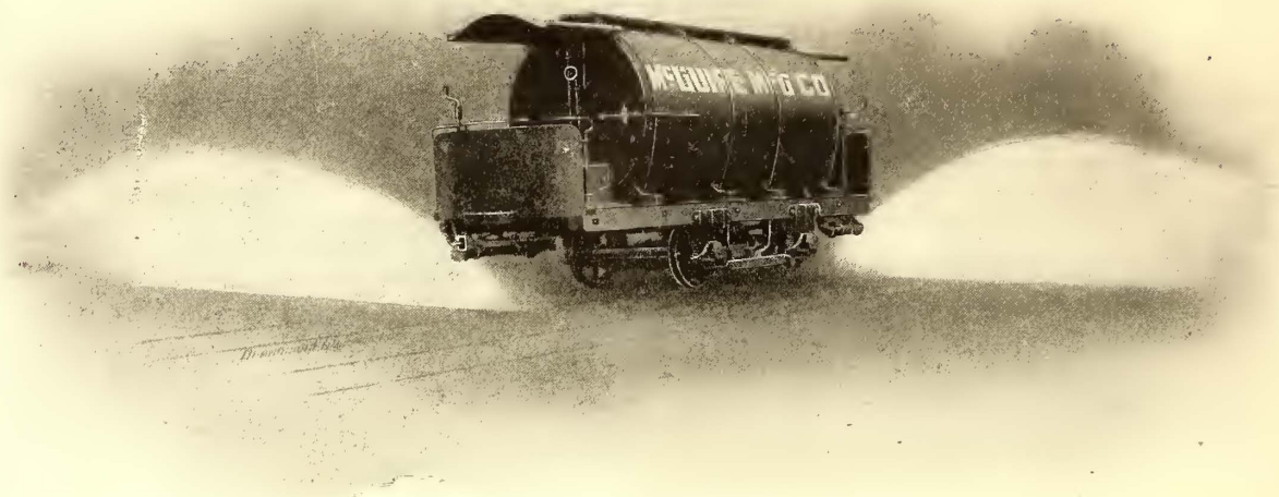
Pneumatic Sprinkler in Operation, Spraying Water 45 Feet on Each Side of Track
