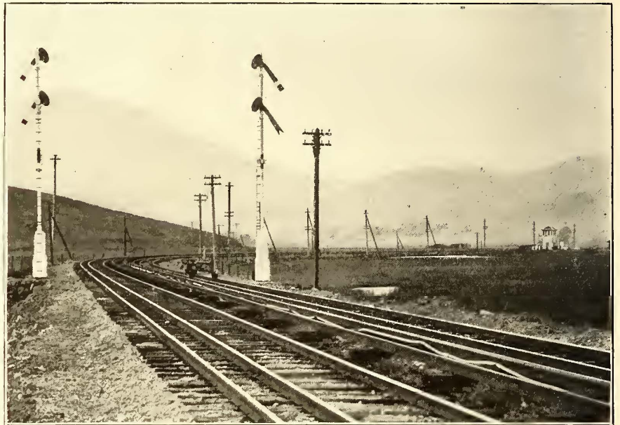
SIGNALS GOVERNING MILL VALLEY JUNCTION, AND INTERLOCKING TOWER AT RIGHT
