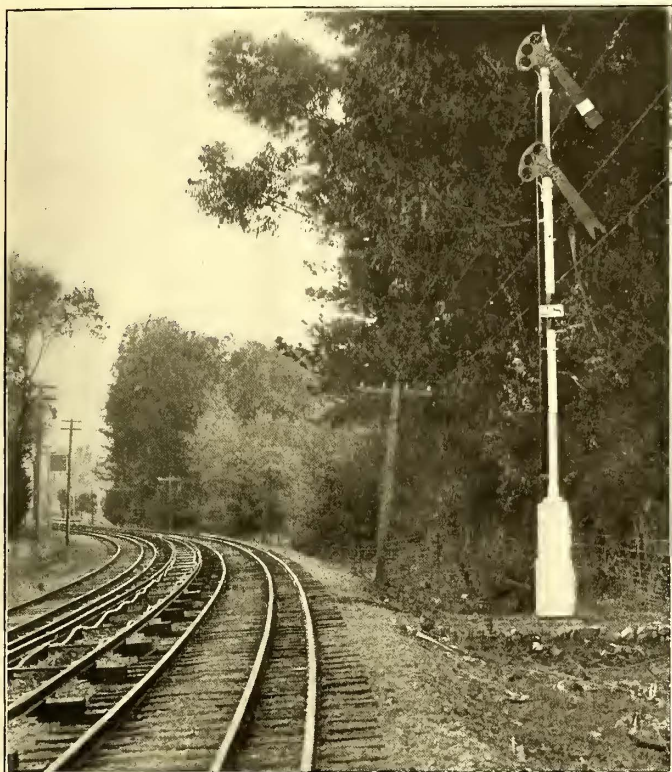
TYPICAL VIEW SHOWING SIGNAL SYSTEM AND METHOD OF LAYING CONTACT-RAIL ON CURVE
