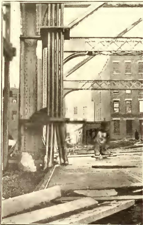
FIG. 1.—OUTLET PIPES, SHOWING METHOD OF ATTACHMENT TO PILLAR
