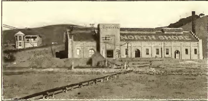
ALTO POWER HOUSE, RETURN TRACK FEEDER IN TROUGH IN GROUND
