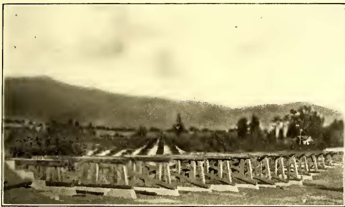
FIG. 22.—STANDARD POST TRESTLE WITHOUT FLOOR
