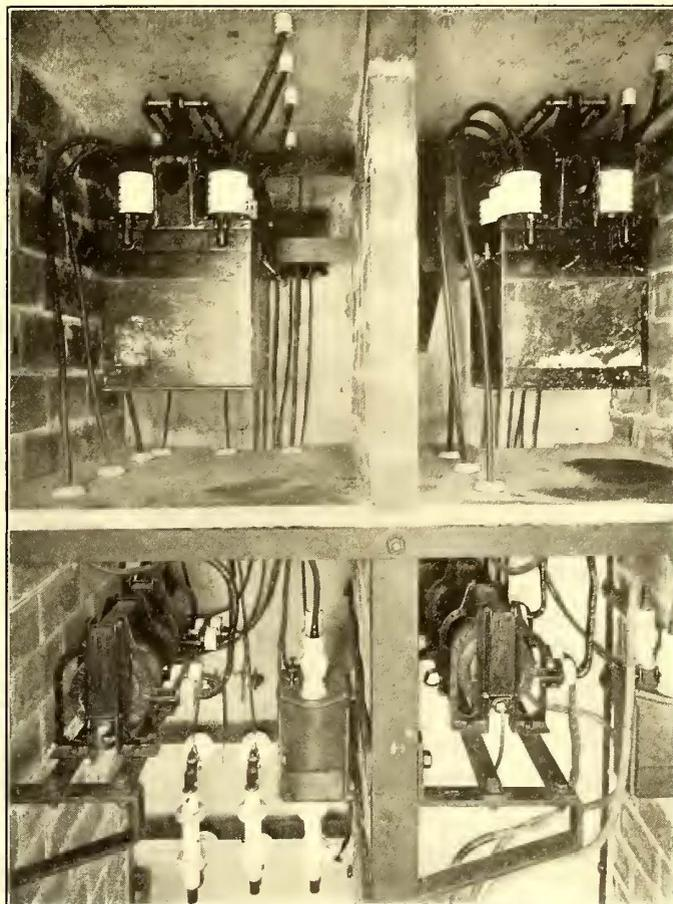
FIG. 15.—HIGH-TENSION OIL SWITCHES IN BRICK CELLS AT LAXEY POWER STATION
