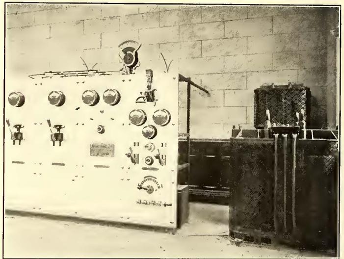
FIG. 12.—BALLAGLASS SWITCHBOARD
