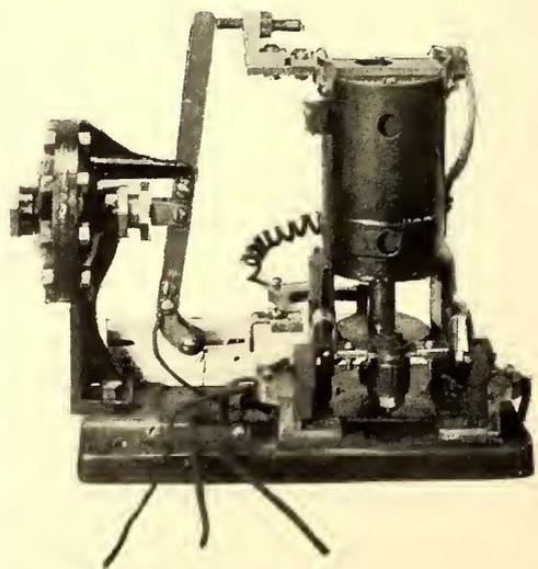
FIG. 3.—AUTOMATIC CUT-OFF WITH COVER REMOVED
