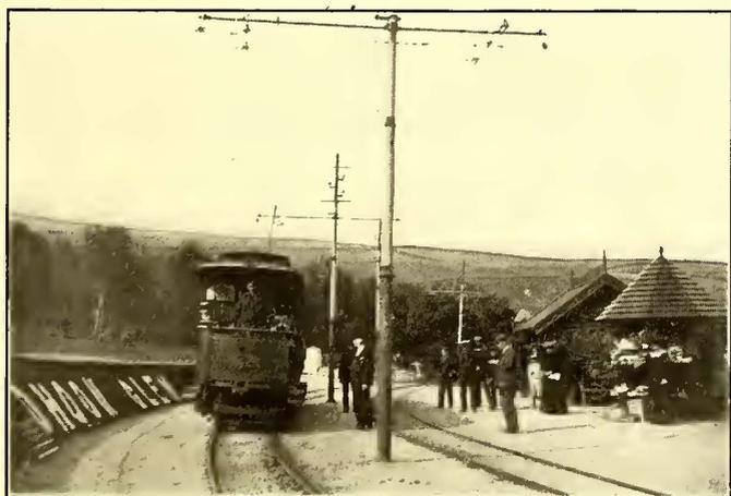
FIG. 16.—TYPICAL OVERHEAD CONSTRUCTION
