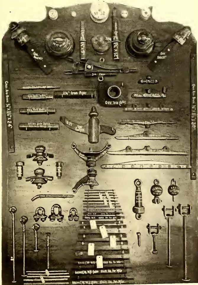
FIG. 1.—STANDARD OVERHEAD LINE APPLIANCES, PACIFIC ELECTRIC RAILWAY
