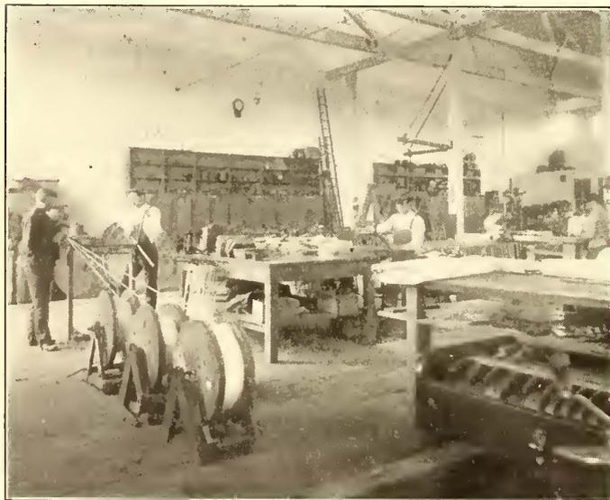
FIG. 6.—ARMATURE SHOP, SHOWING ARMATURE COIL WINDING
