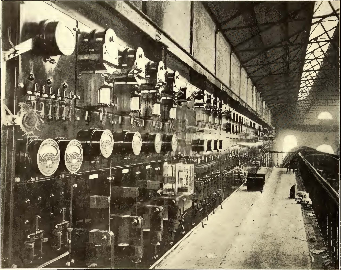
VIEW OF SWITCHBOARD GALLERY, MAIN POWER STATION
