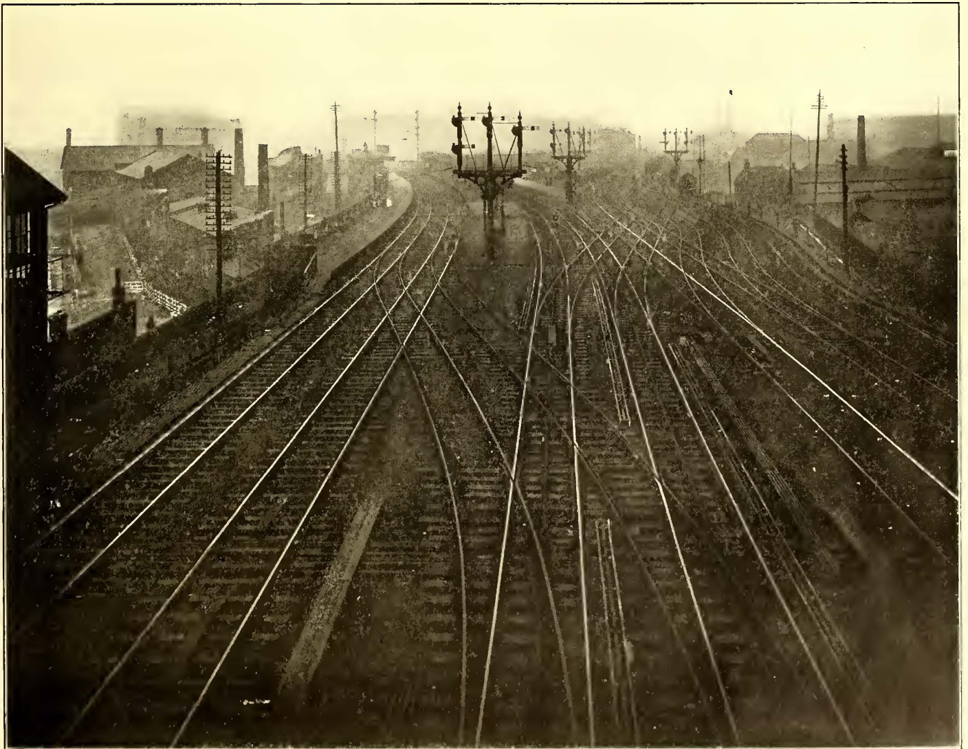
VIEW AT SANDHILLS, SHOWING JUNCTION OF ELECTRIC AND STEAM RAILROAD DIVISIONS
