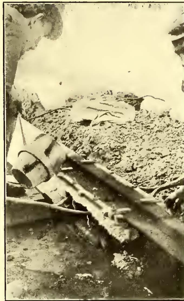
FIG. 5.—POURING A JOINT WITH MOLTEN ZINC
