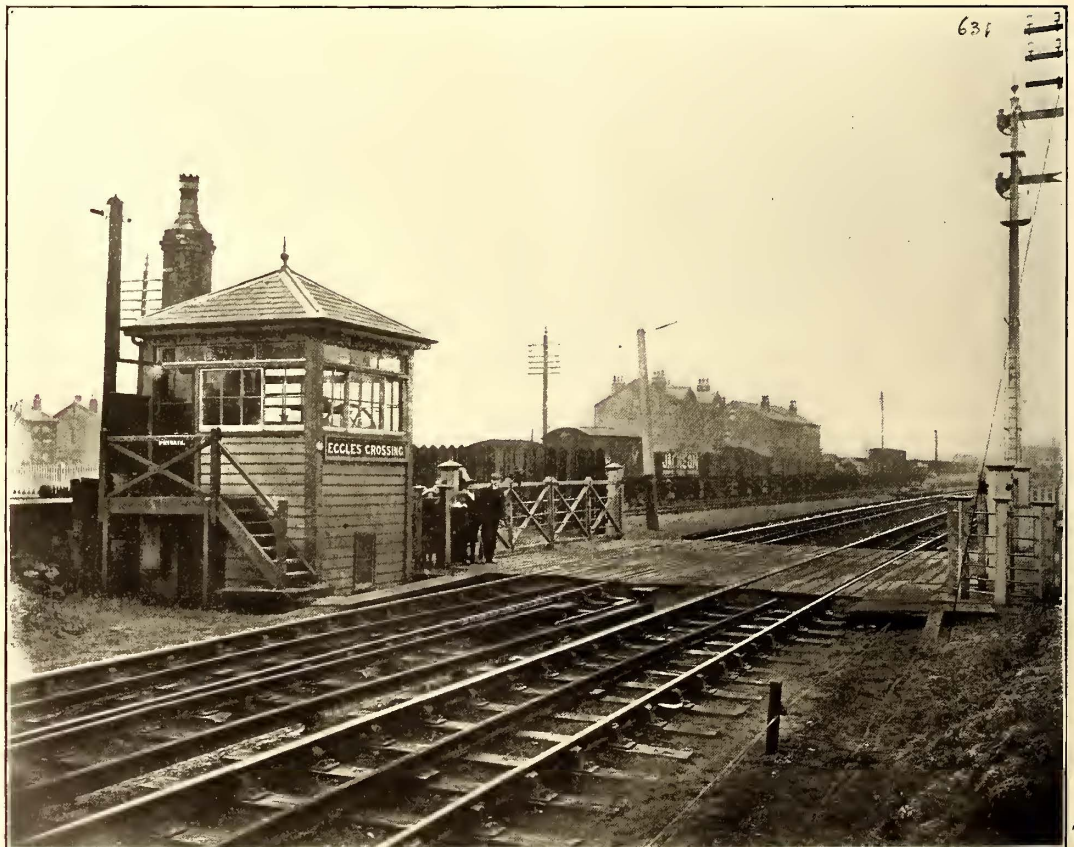
VIEW AT GRADE CROSSING, SHOWING THIRD AND FOURTH RAIL INCLINES, THE FORMER PROTECTED BY GUARDS
