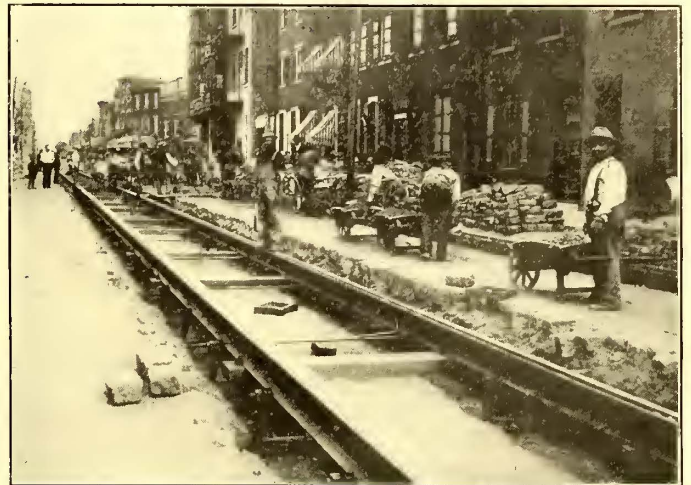
FIG. 11.—VIEW AFTER THE U-SHAPED TIE RODS ARE FASTENED TO THE RAILS
