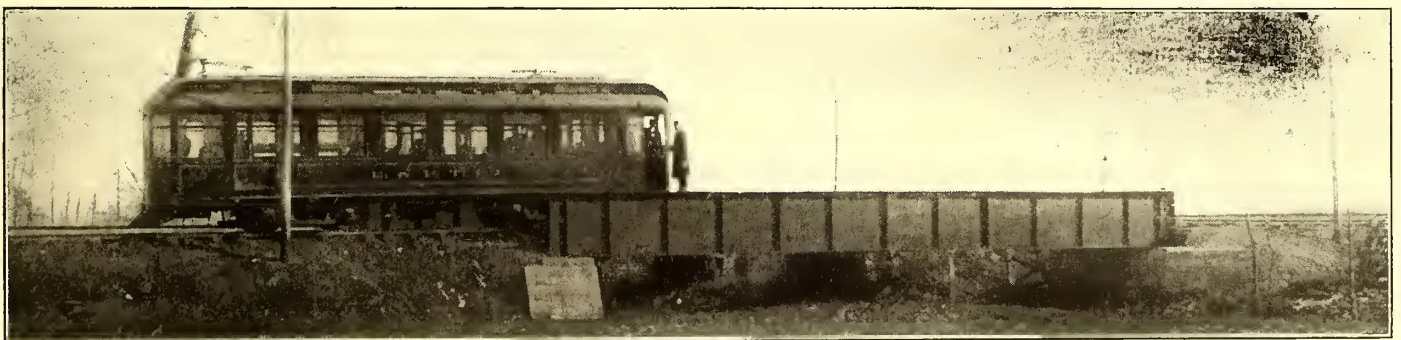
PLATE GIRDER BRIDGE
