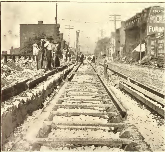
VIEWS OF FORBES STREET, PITTSBURG, SHOWING METHOD OF LAYING STEEL TRACK STRUCTURE IN PAVED STREET
