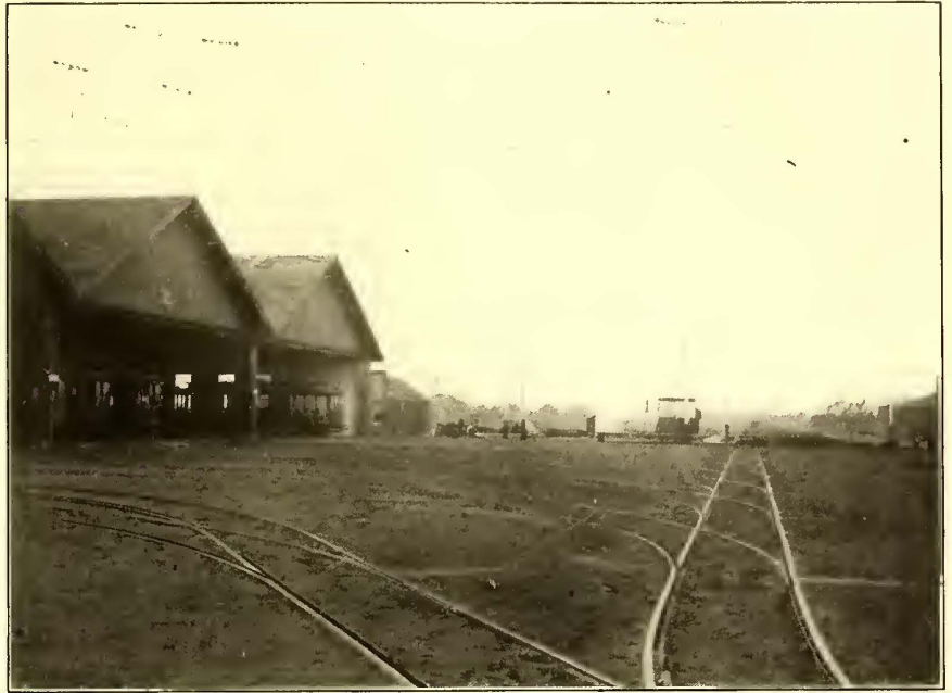
FIG. 12.—EAST END OF CAR HOUSE, SHOWING SPECIAL TRACK AND OVERHEAD WORK
