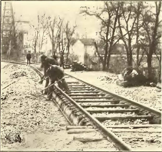
ALL STEEL STRUCTURE ON EXPOSED TRACK
