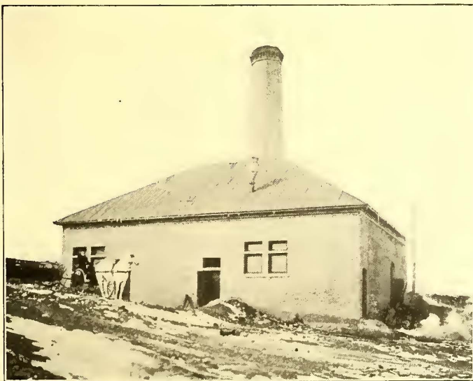
FIG. 1.—EXTERIOR OF POWER STATION
