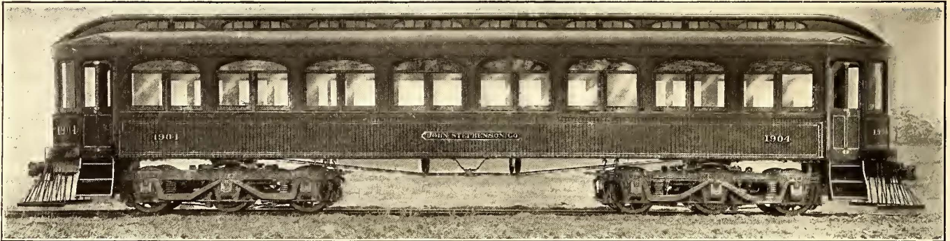
VIEW SHOWING SIX-WHEEL TRUCKS, DOUBLE VESTIBULES, ROOF CONSTRUCTION AND OTHER EXTERIOR DETAILS
