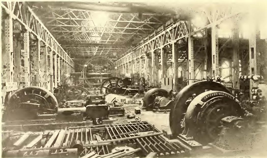
GENERAL VIEW IN MACHINERY HALL
