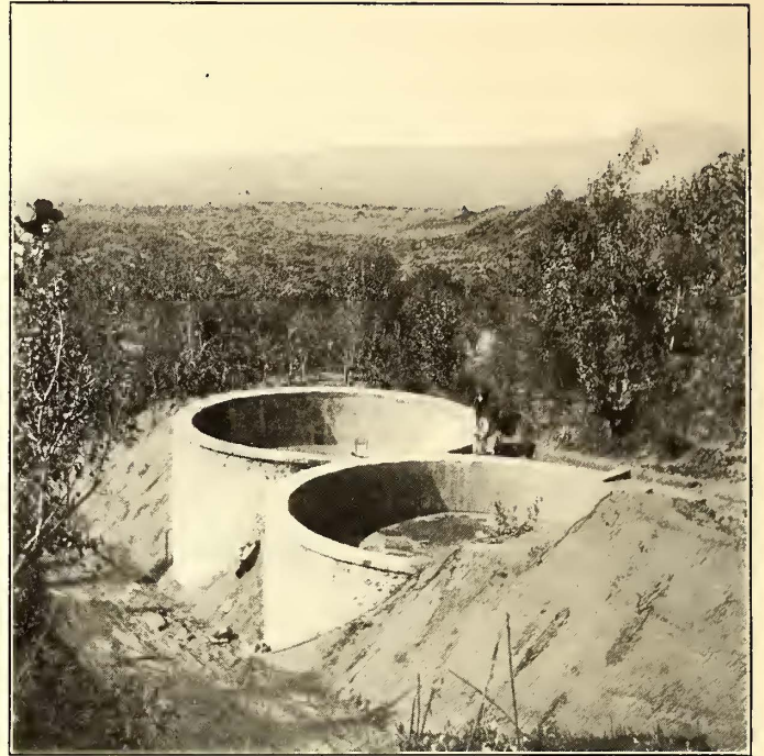
RESERVOIRS FOR RAIN WATER
