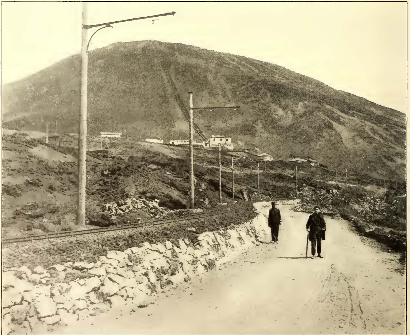
APPROACH TO THE LOWER STATION OF THE CABLE RAILWAY
