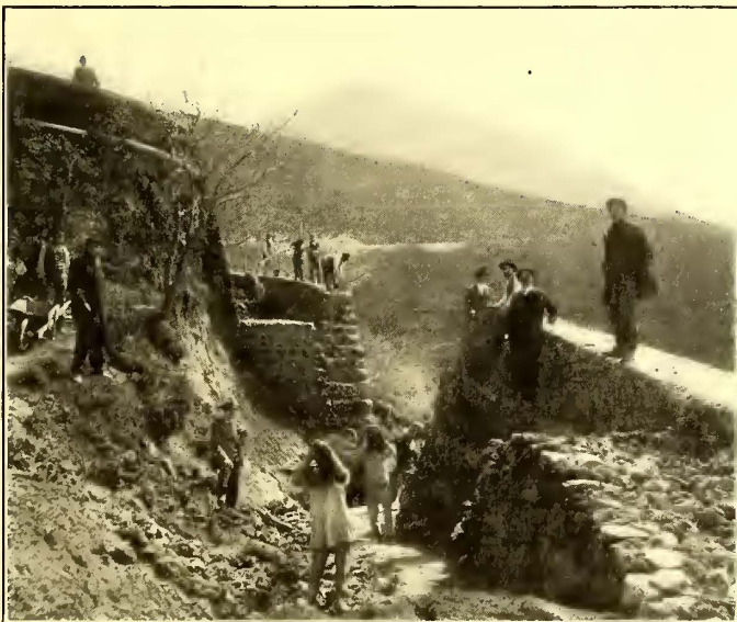
BUILDING THE SUPPORTING WALL BENEATH THE TERRACE OF THE OBSERVATORY
