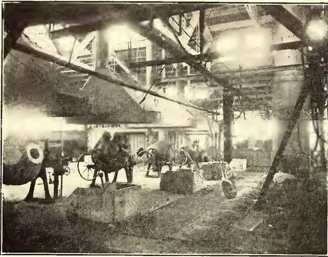
FIG. 1.—PART OF BRASS FOUNDRY, SHOWING GAS FURNACES
