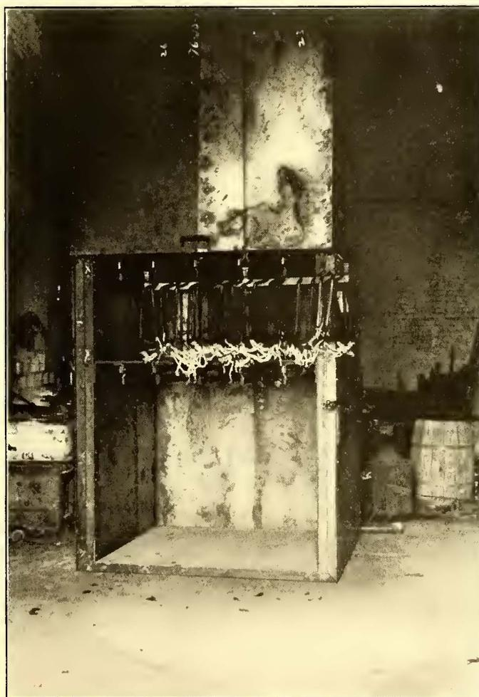
FIG. 12.—BAKING OVEN, WITH RACK OF COILS PULLED OUT
