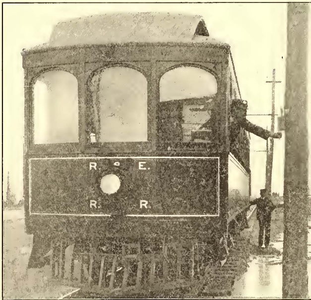
FIG. 1.—MOTORMAN PLUGGING CONNECTION TO TELEPHONE JACK BOX ON POLE
