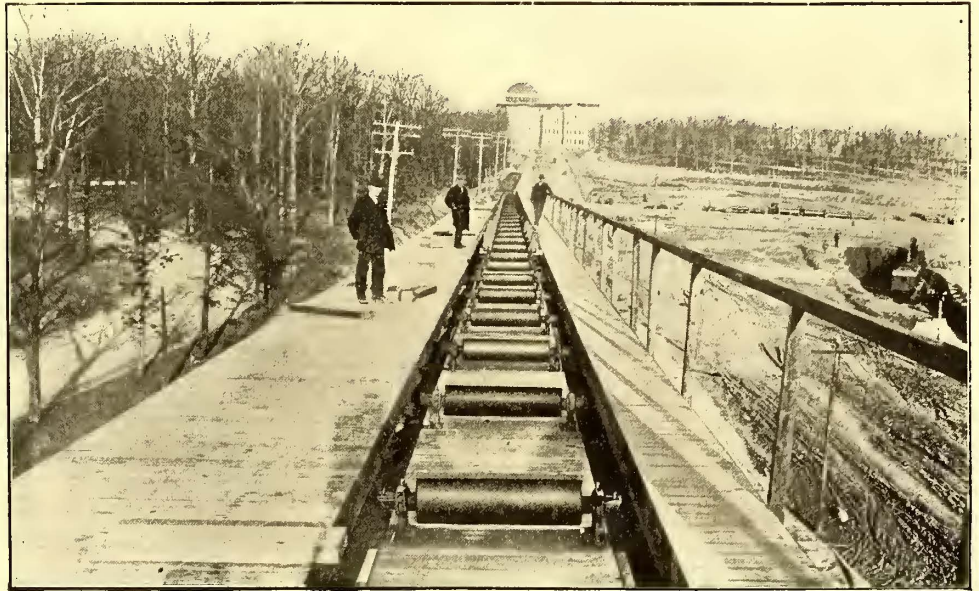
FIG. 1.—CARRIERS USED IN TWO-BELT CONVEYOR.
