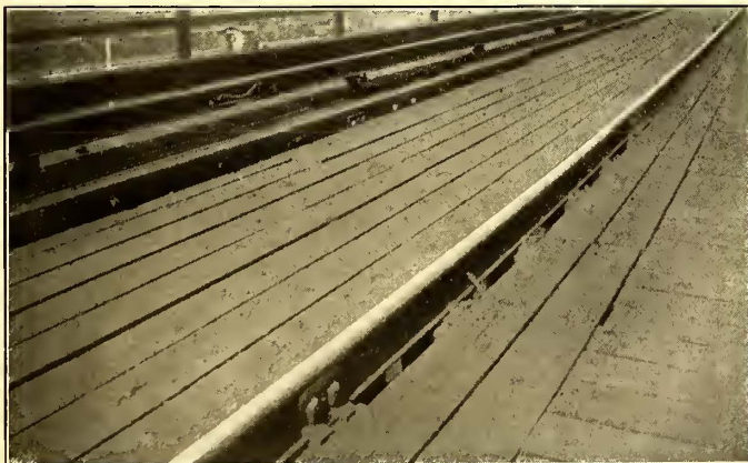
FIG. 9.—TRACK ON SOUTH END OF TRIANGULAR JUNCTION
