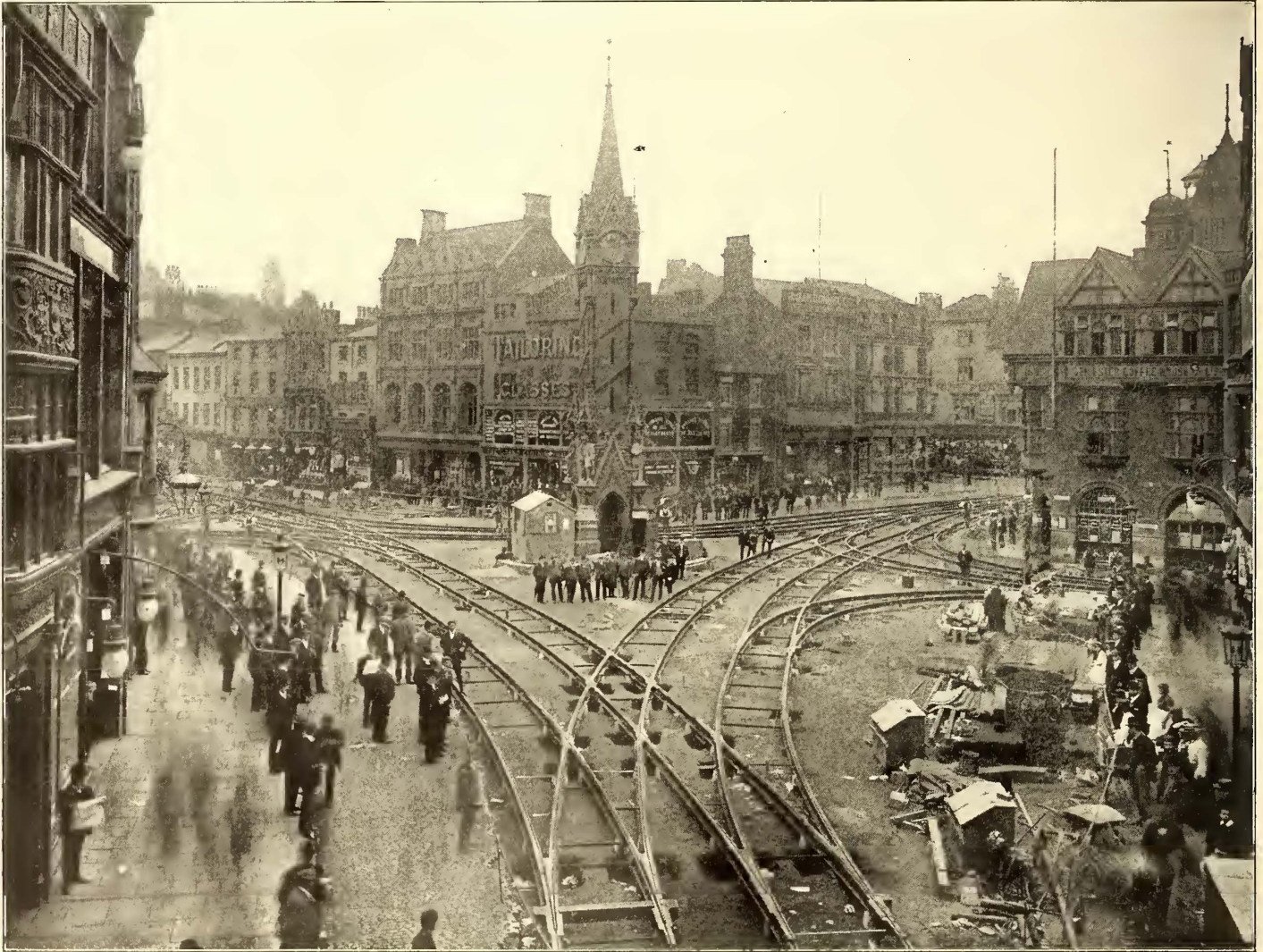
LEICESTER TRAMWAYS—CLOCK TOWER JUNCTION, SHOWING SPECIAL WORK
