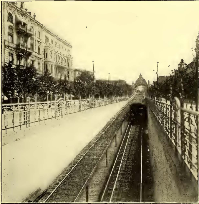
FIG. 15.—INCLINE ON KLEIST STRASSE BETWEEN SUBWAY AND ELEVATED
