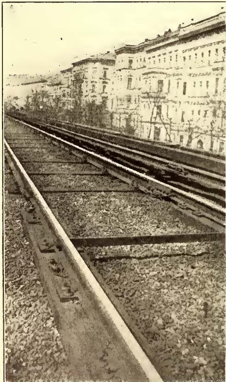
FIG. 2.—STRINGERS ON EASTERN SECTION
