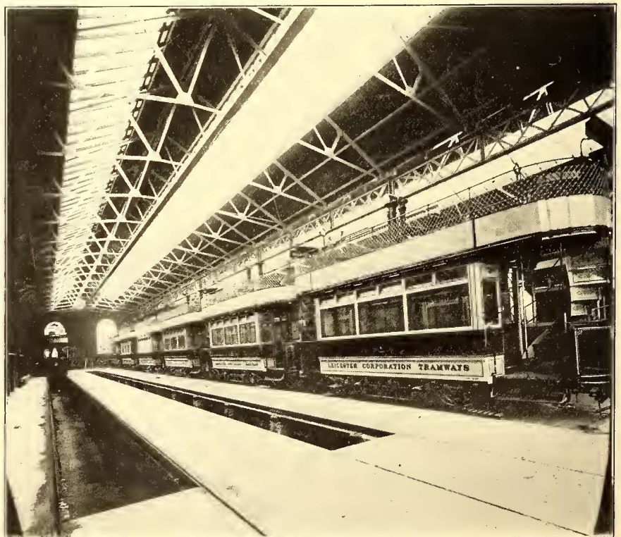
MAIN CAR DEPOT—ABBEY PARK ROAD
