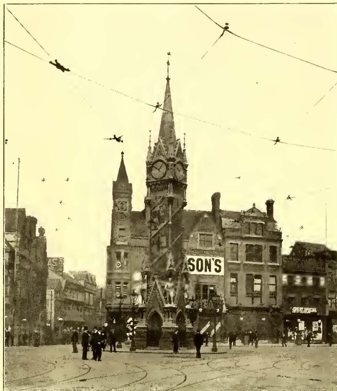
COMPLICATED OVERHEAD EQUIPMENT AND SPECIAL WORK AT CLOCK TOWER
