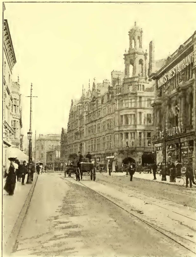
SPAN POLE CONSTRUCTION—GRANBY STREET
