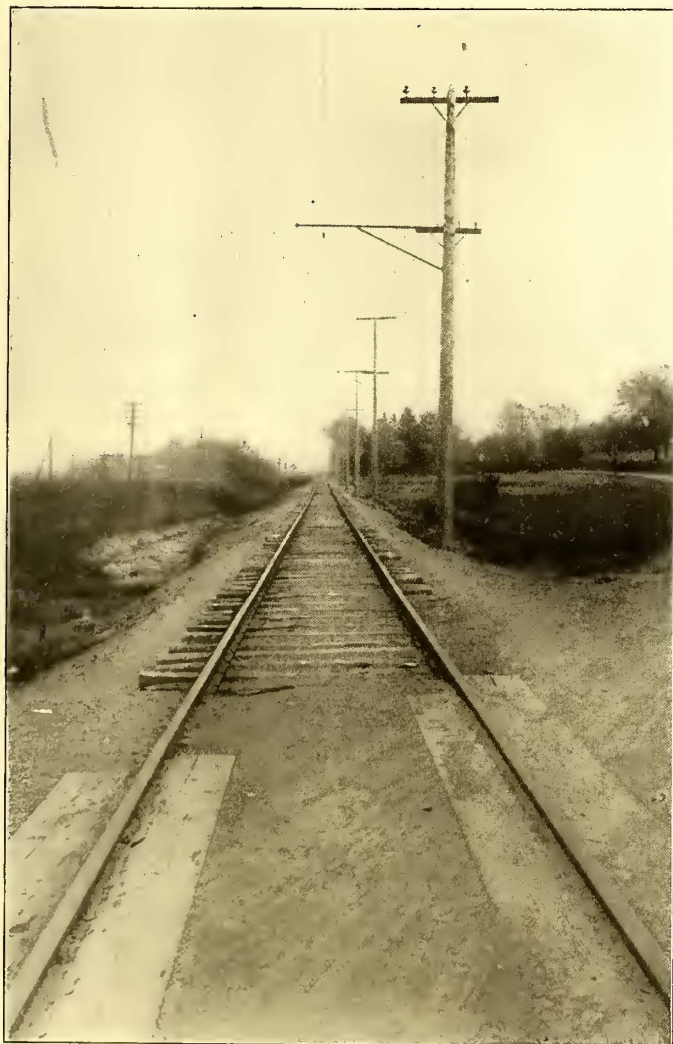
LINE VIEW, SHOWING OVERHEAD CONSTRUCTION
