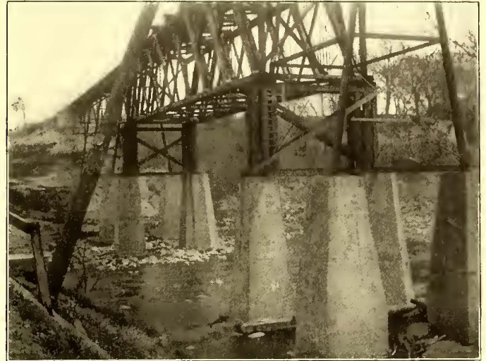
TIMBER SECTION BRIDGE ON CONCRETE PIERS
