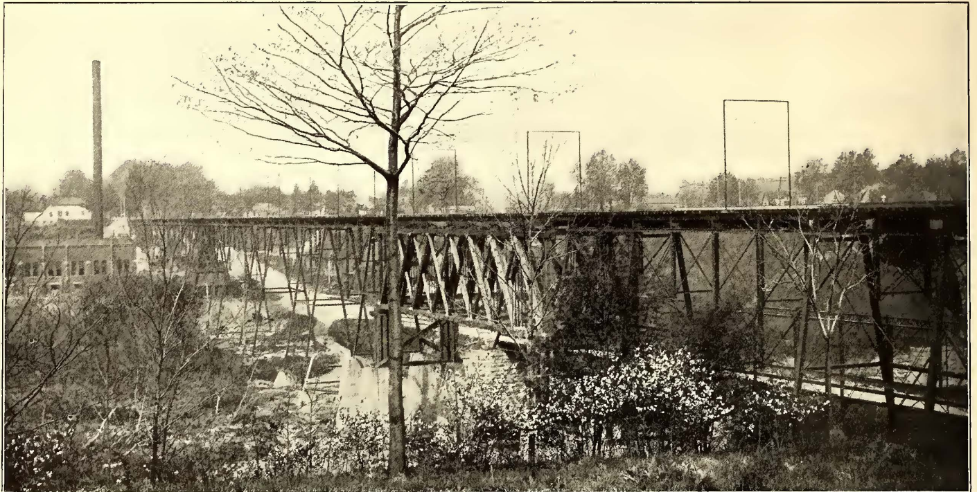
STEEL VIADUCT AT GRAND RIVER
