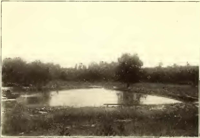
COOLING POND AND SLUICE FOR CONDENSING WATER
