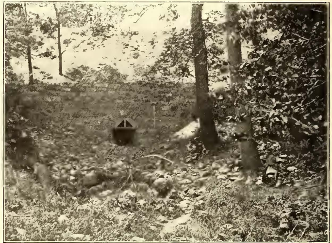
AN EXAMPLE OF MASONRY CONSTRUCTION
