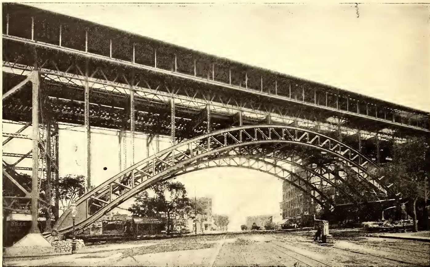
SIDE VIEW OF MANHATTAN VIADUCT
