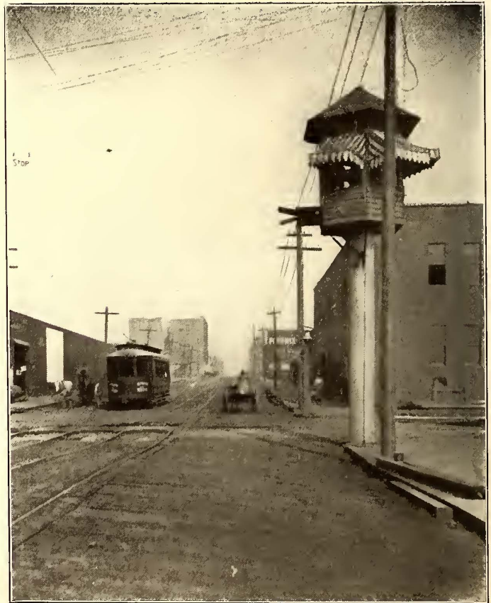
FIG. 37.—DESPATCHER'S TOWER AT SOUTHERN PACIFIC CROSSING
