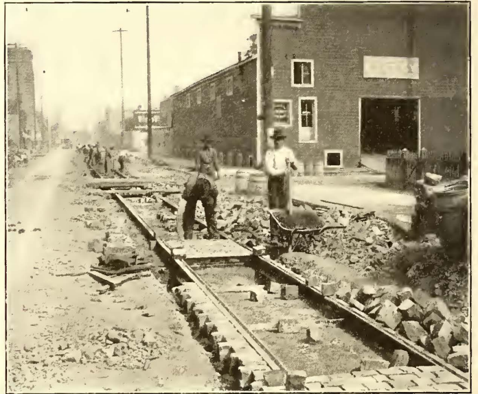
FIG. 14.—PREPARING CEMENT MORTAR AND LAYING BASALT PAVING BLOCKS IN NEW TRACK
