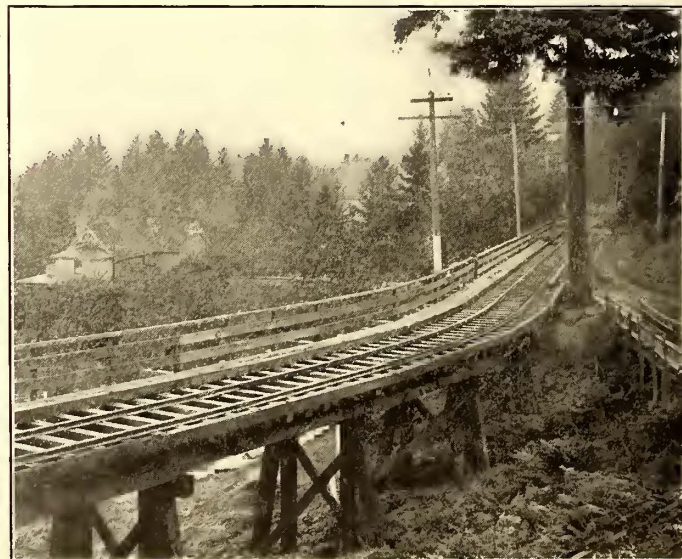
FIG. 8.—WOODEN TRESTLE ON WESTERN SIDE OF LOOP ON PORTLAND HEIGHTS LINE
