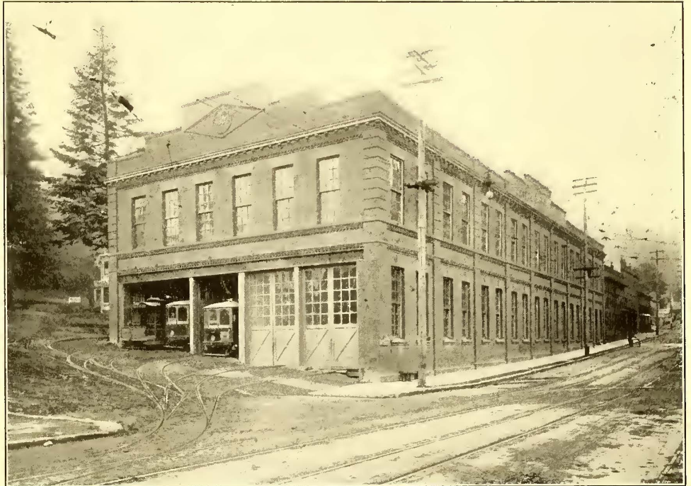
FIG. 28.—REPAIR SHOP AND CAR HOUSES OF PORTLAND RAILWAY COMPANY
