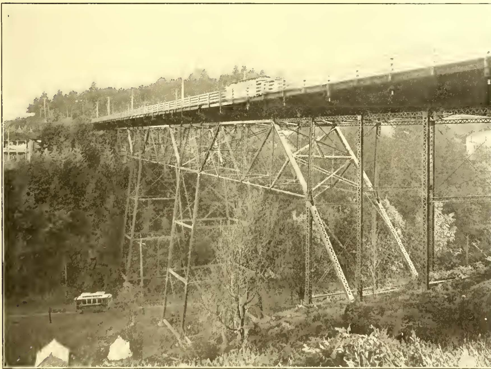
FIG. 4.—FORD STREET STEEL VIADUCT ON PORTLAND HEIGHTS LINE, 117 FT. HIGH AND 560 FT. LONG
