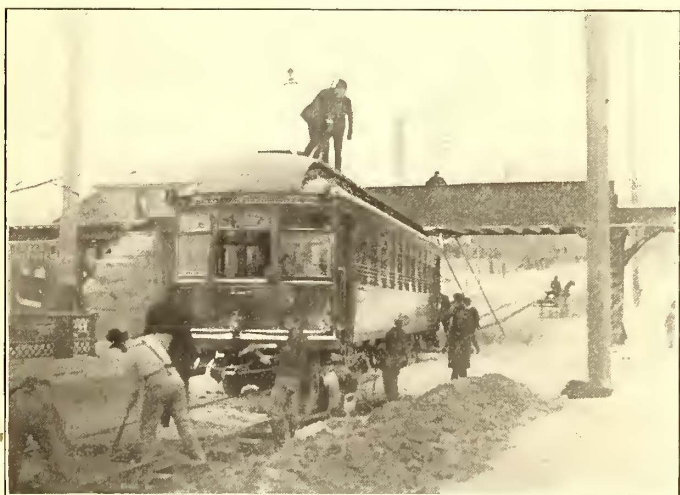
THE BRIDGE THAT SEPARATES INDIANA FROM OHIO. INDIANAPOLIS & EASTERN SPECIAL CAR GOING OVER OHIO LINES. TROLLEY BEING REMOVED.
