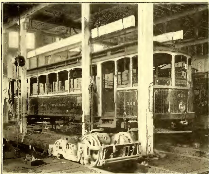
FIG. 23.—VIEW IN REPAIR SHOP, SHOWING SLING CAR HOIST AND STANDARD MAXIMUM TRACTION TRUCK
