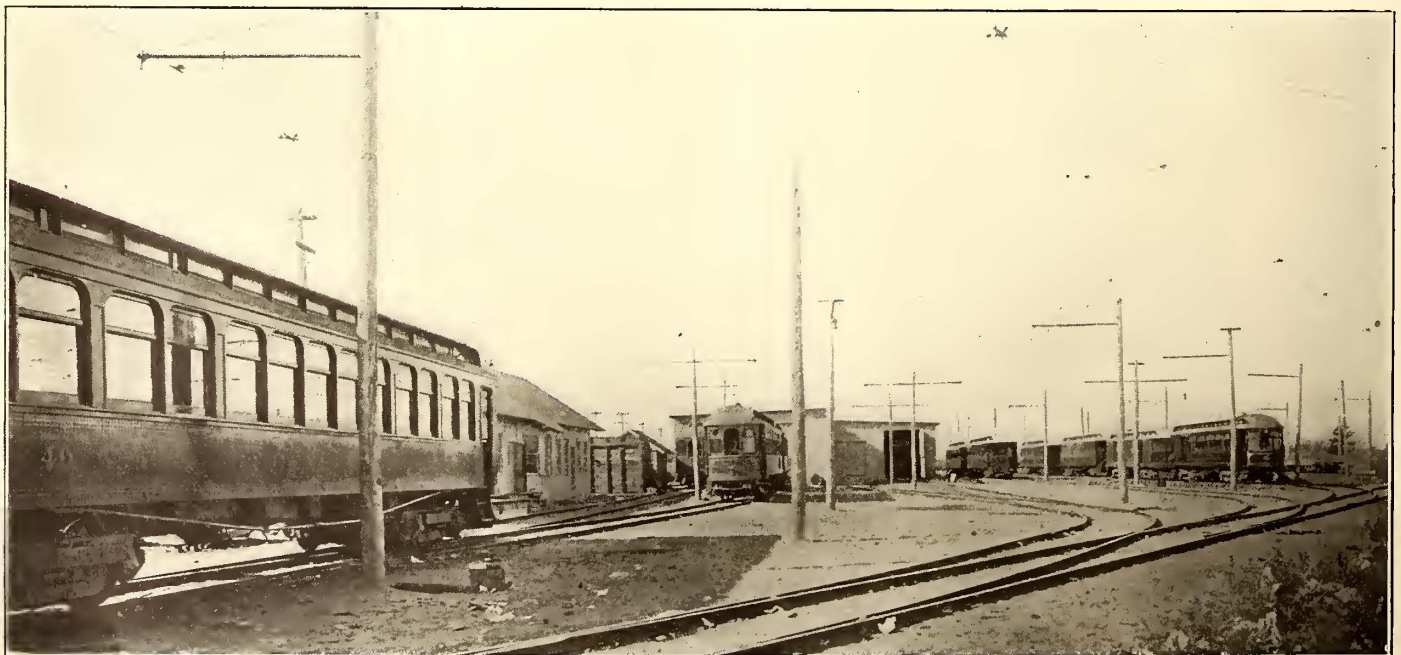
THE ARRANGEMENT OF STORAGE AND REPAIR TRACKS IN THE SHOP YARD AT ALBION, SHOWING SHOP BUILDINGS IN BACKGROUND
