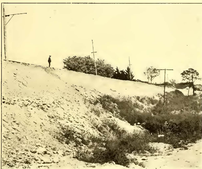
A HEAVY FILL ON THE STARK ELECTRIC RAILWAY
