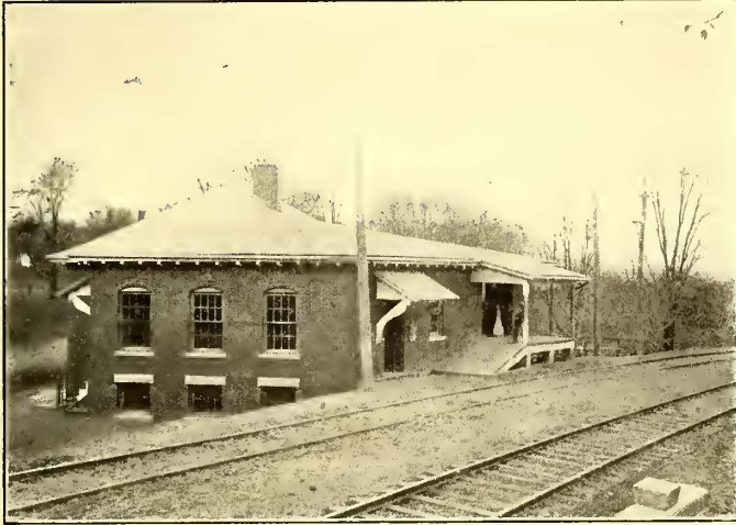
THE DAMASCUS SUB-STATION
