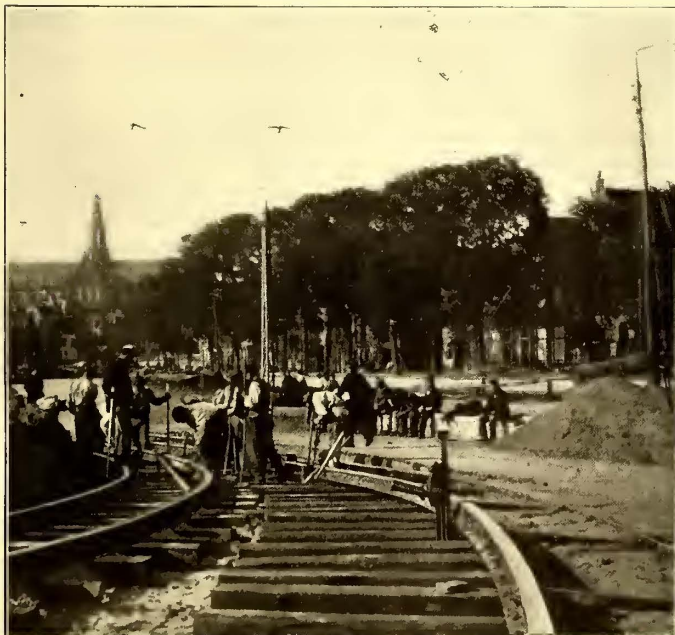
VIEW SHOWING METHOD OF LAYING TRACK
