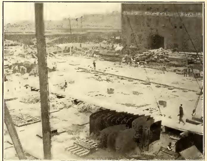
LAYING THE CONCRETE FOR THE STATION FOUNDATION
