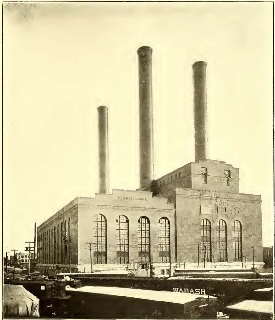
VIEW OF POWER STATION OF LONG ISLAND RAILROAD COMPANY FROM FREIGHT YARDS
