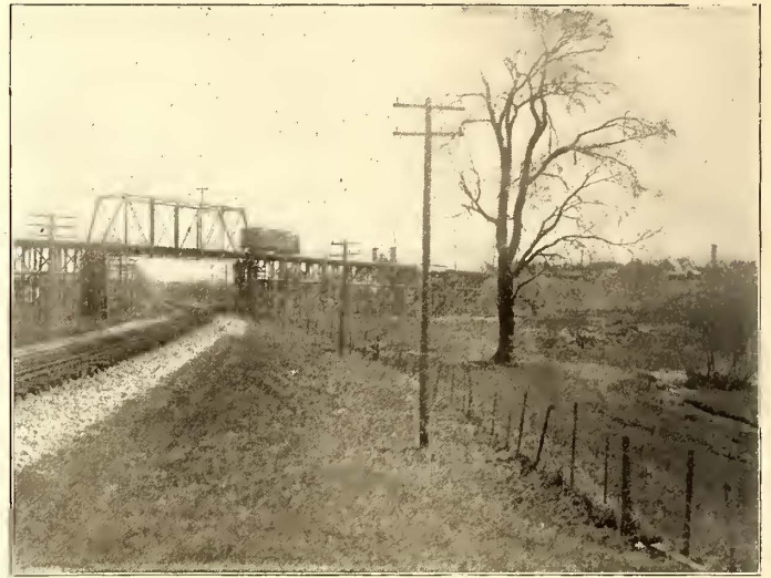
CROSSING ABOVE THE PENNSYLVANIA RAILROAD AT LOUISVILLE
