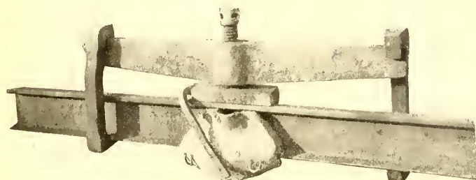
FIG. 3.—MOLDS AND CLAMPS READY TO WELD, POURING SIDE
