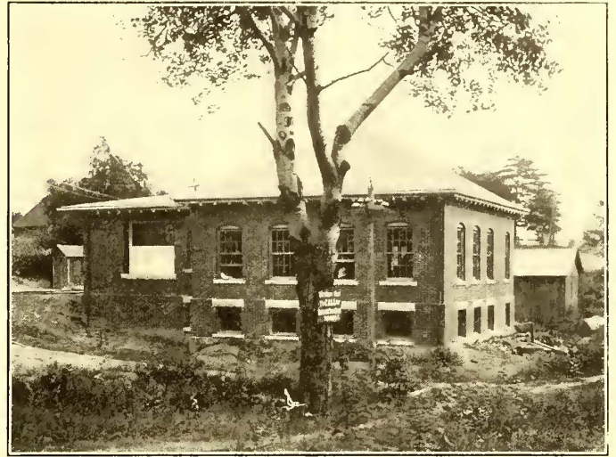
THE LOUISVILLE SUB-STATION
