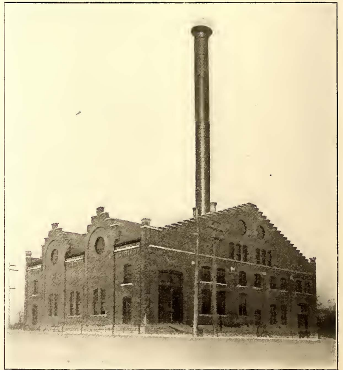
EXTERIOR OF POWER HOUSE
