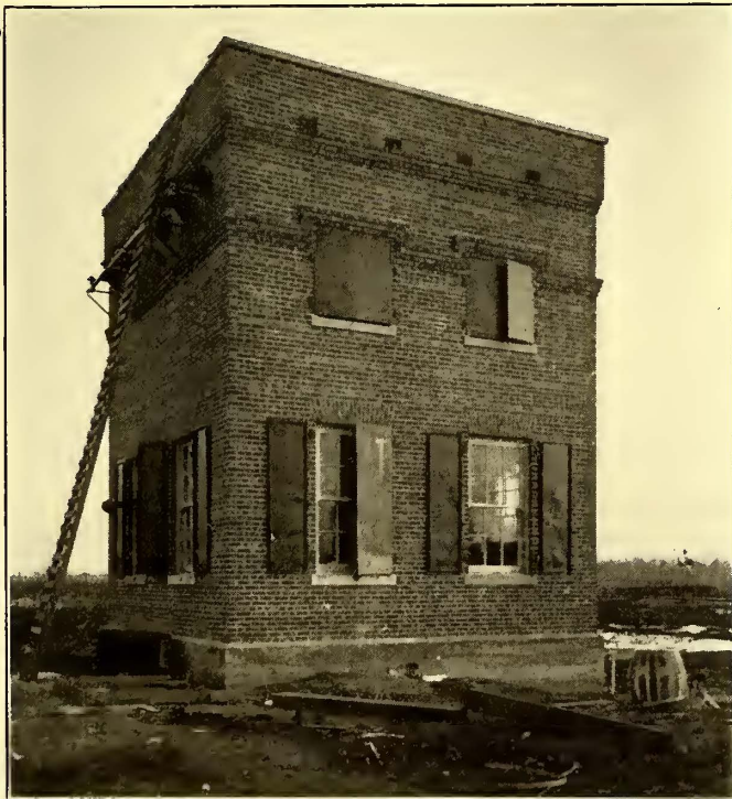
TRANSFORMER STATION AT REEDVILLE, IND.
