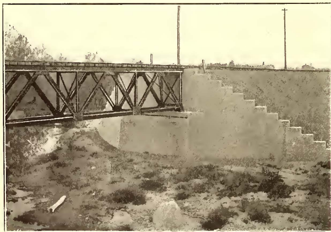
BRIDGE 105 FT. LONG OVER BIG SUGAR CREEK, NEAR NEW PALESTINE, IND.
