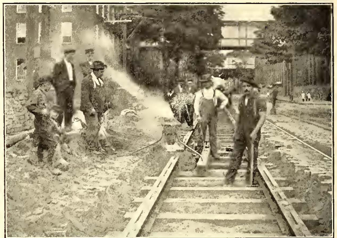
THERMIT REACTION IN PROGRESS
