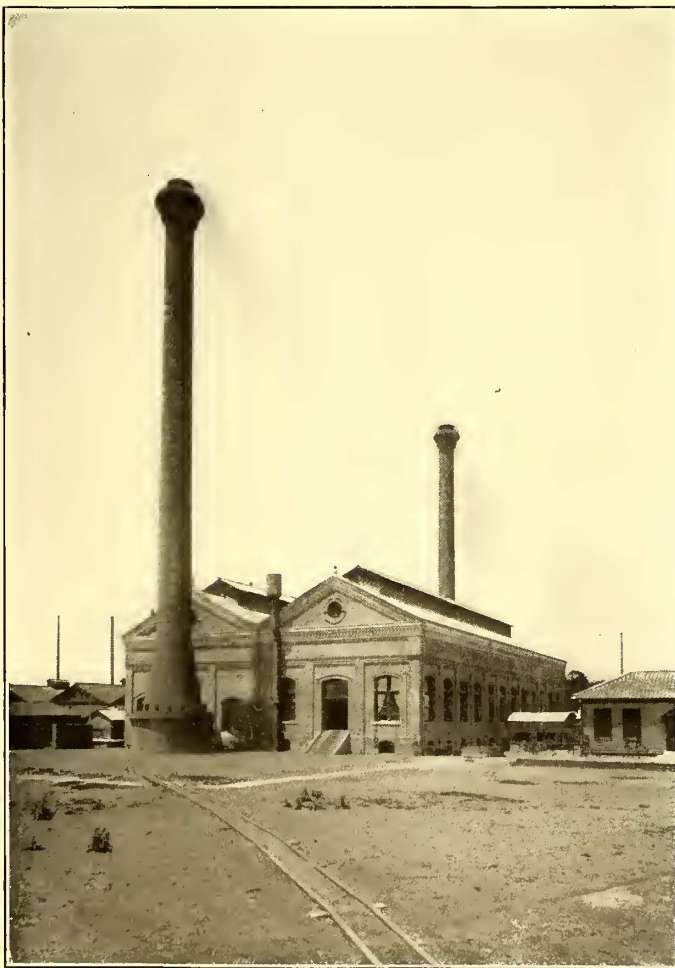
AN EXTERIOR VIEW OF THE POWER STATION
