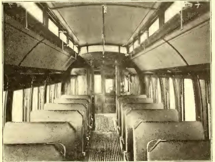
SEATING ARRANGEMENT OF BLOOMINGTON, PONTIAC & JOLIET INTERURBAN CAR
