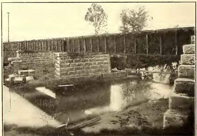
BRIDGE OVER BLUE RIVER, NEAR MORRISTOWN, IND.
