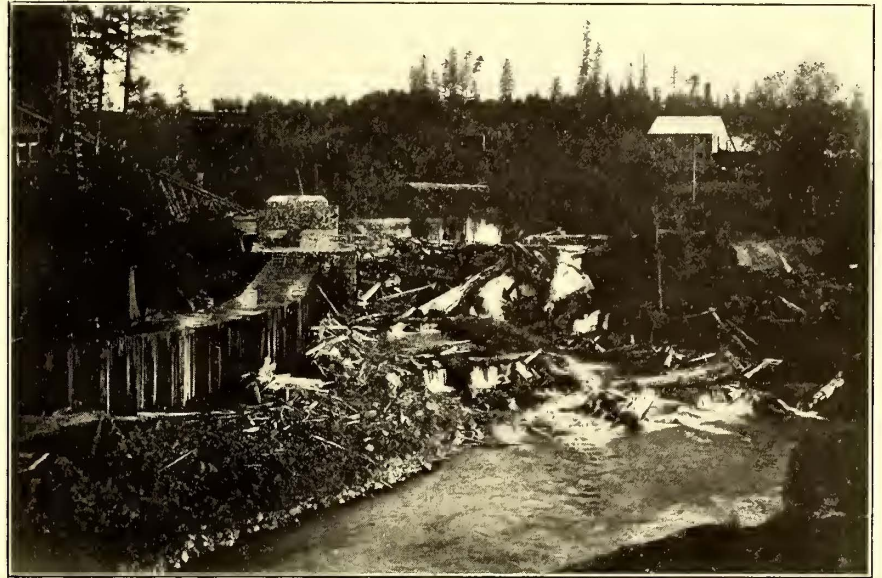
DAM, INTAKE AND SQUARE WOODEN FLUME OF OLYMPIA PLANT
