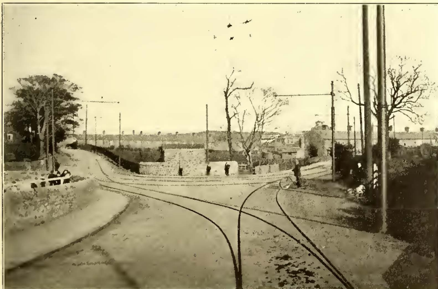
A TRACK SWITCH IN SUNDERLAND, SHOWING ALSO THE TYPE OF OVERHEAD CONSTRUCTION
