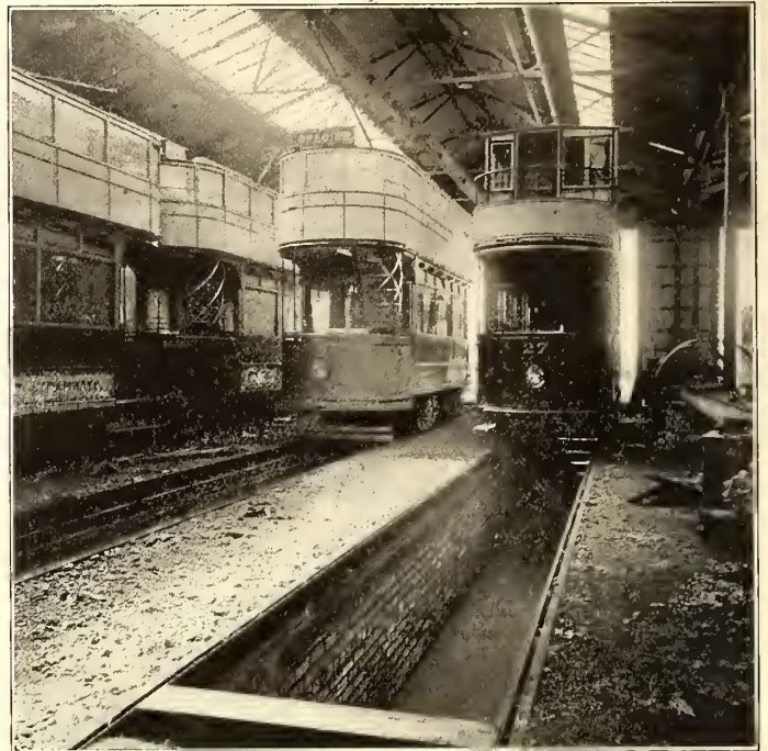
A VIEW OF THE CAR HOUSE INTERIOR
