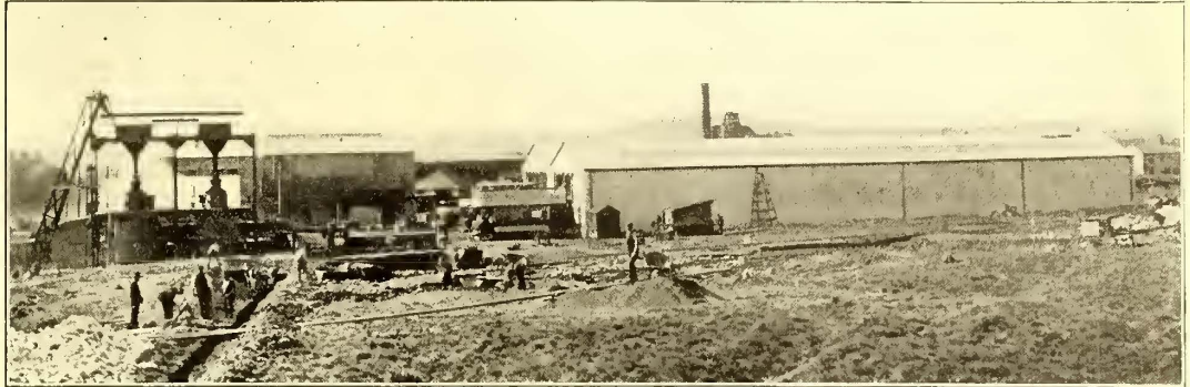
VIEW SHOWING LOCATION OF GAS PRODUCER PLANT IN FRONT OF THE CAR SHEDS
