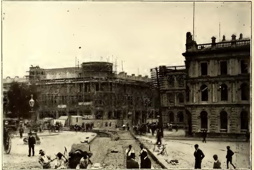
MAKING EXCAVATIONS FOR THE TRACKWORK IN CATHEDRAL SQUARE, CHRISTCHURCH
