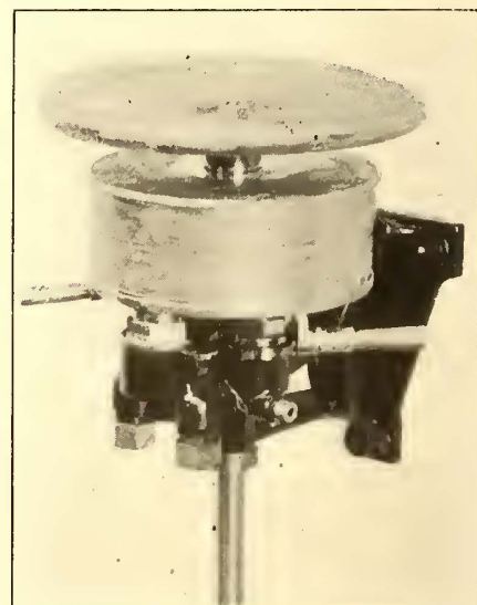
FIG. 20.—MASTER CONTROLLER OF THIRD LOCOMOTIVE
