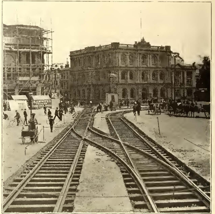
LAYING PERMANENT WAY AT CATHEDRAL SQUARE, CHRISTCHURCH
