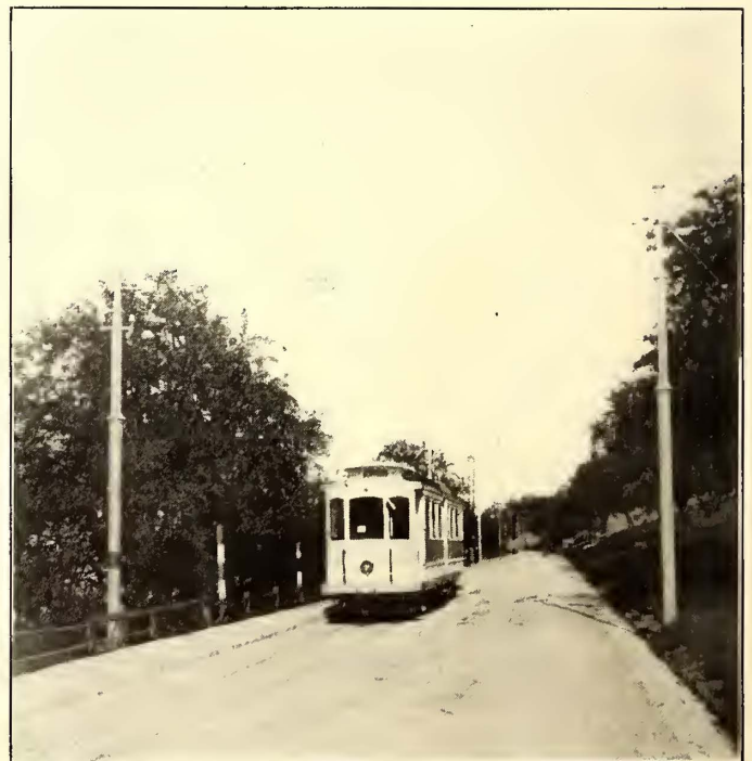
JUNCTION POINT OF THE 800 AND 500-VOLT TROLLEYS, SHOWING EXTRA OVERHEAD WIRE
