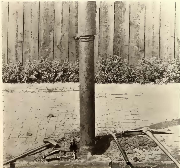
Pole with Old Concrete Removed Prior to Slipping on Sleeve
