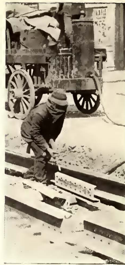
Sand Blasting Rail Ends and Plates
