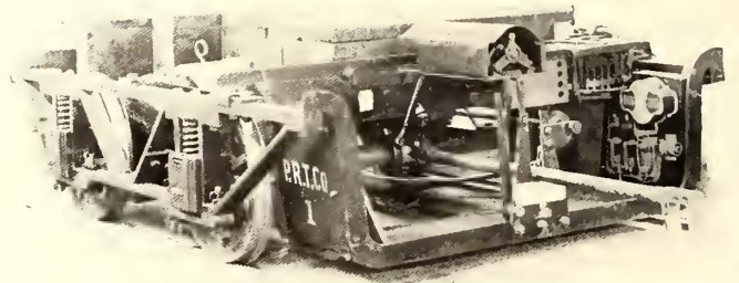
REAR VIEW OF STORAGE BATTERY LOCOMOTIVE FOR SHIFTING TRUCKS IN SHOPS
