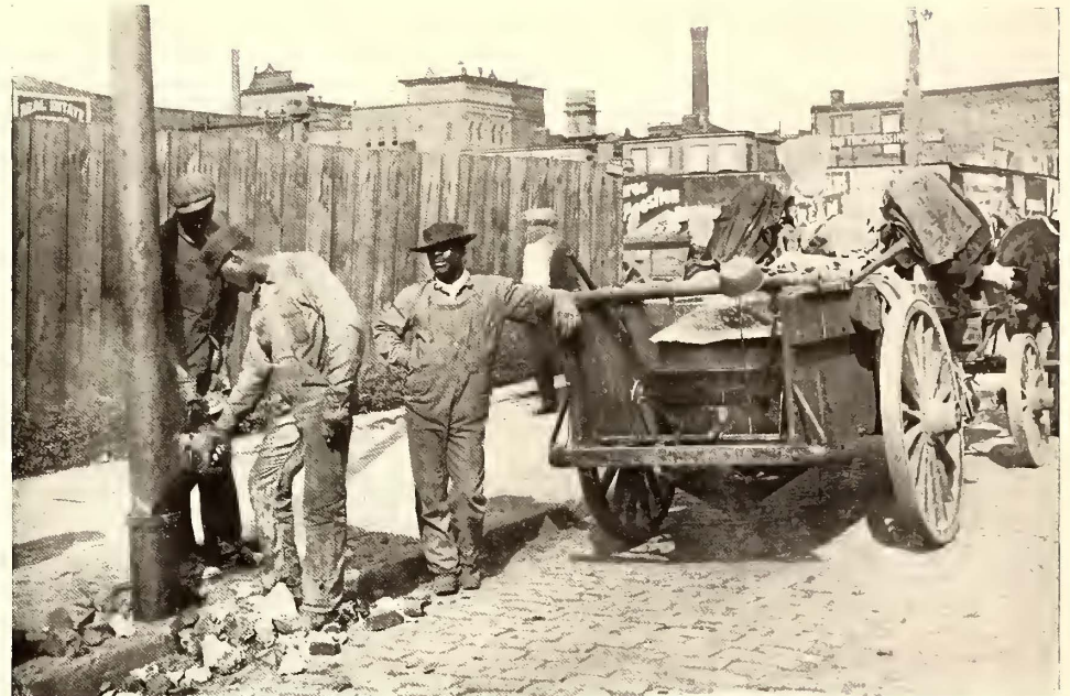
Pouring the Sulphur—Wagon for Melting Sulphur at Right
