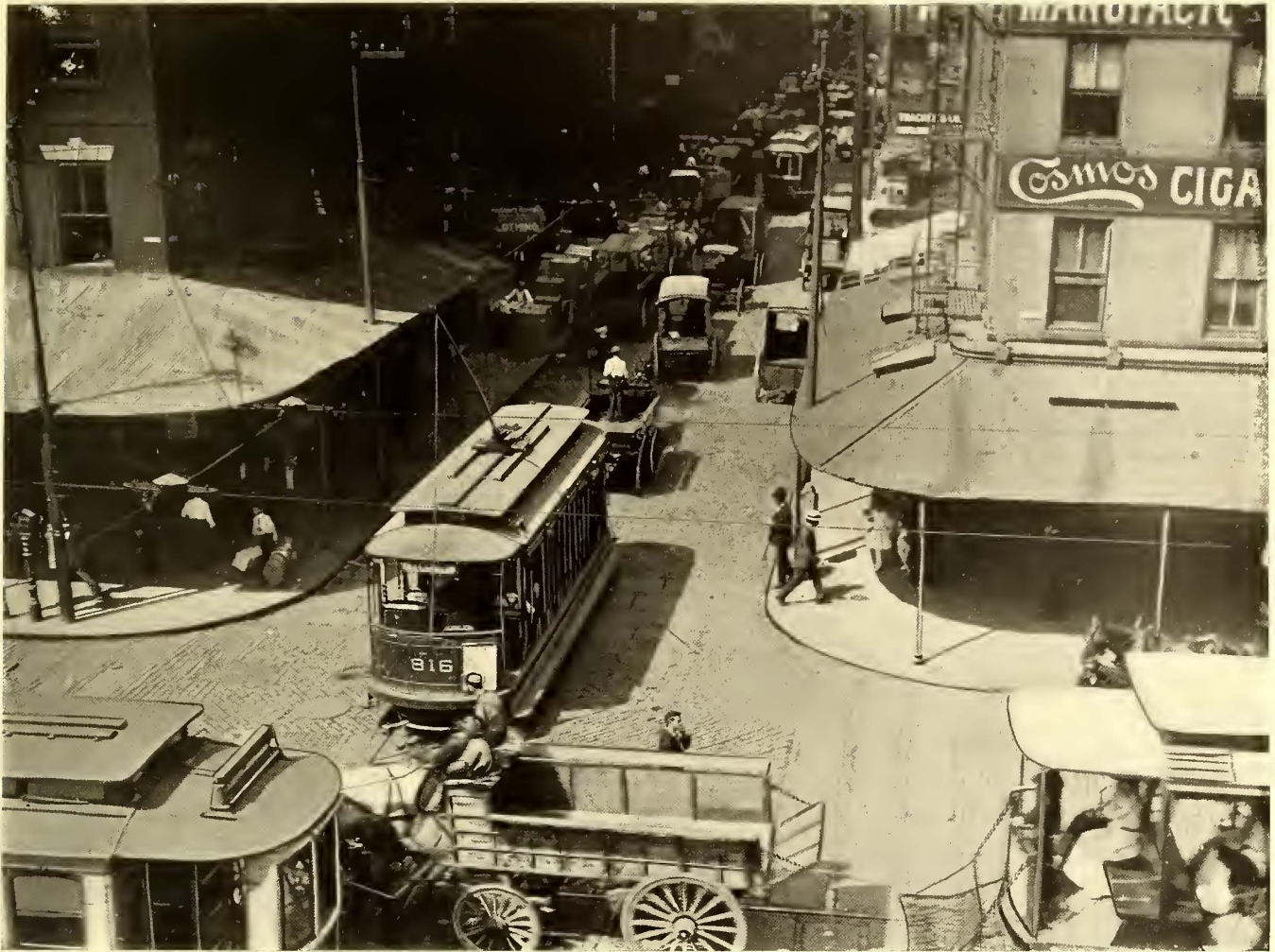
INTERSECTION OF THIRD AND MARKET STREETS, LOOKING NORTH ON THIRD STREET.—THE VIEW SHOWS THE STREET CONGESTION ON AN ORDINARY AFTERNOON
