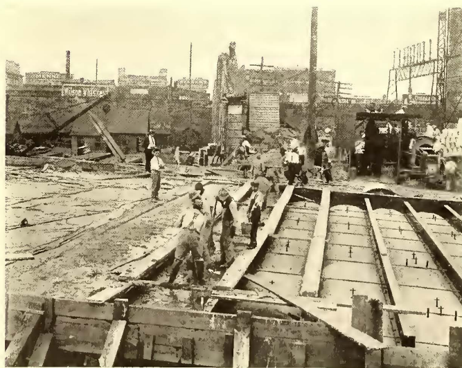
VIEW SHOWING SUBWAY ROOF CONSTRUCTION
