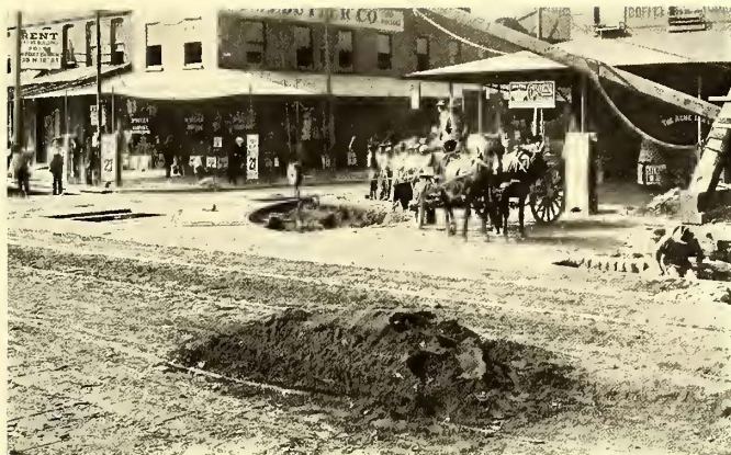
COMMENCING EXCAVATION WORK ON SUBWAY TRENCH
