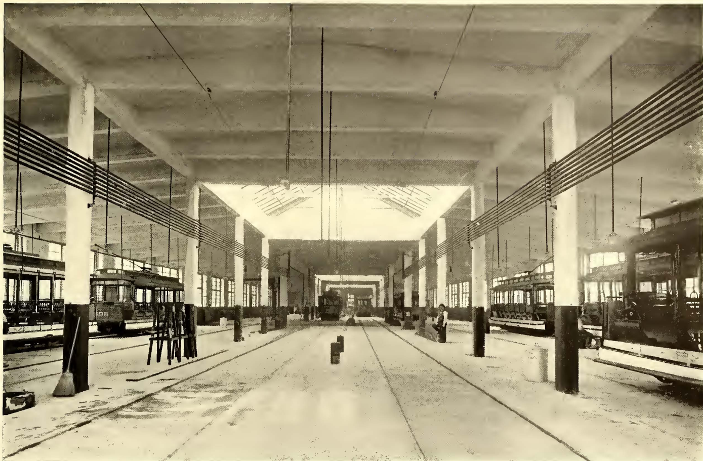
PAINT ROOM, NEW CONCRETE ADDITION TO KENSINGTON AVENUE SHOPS
