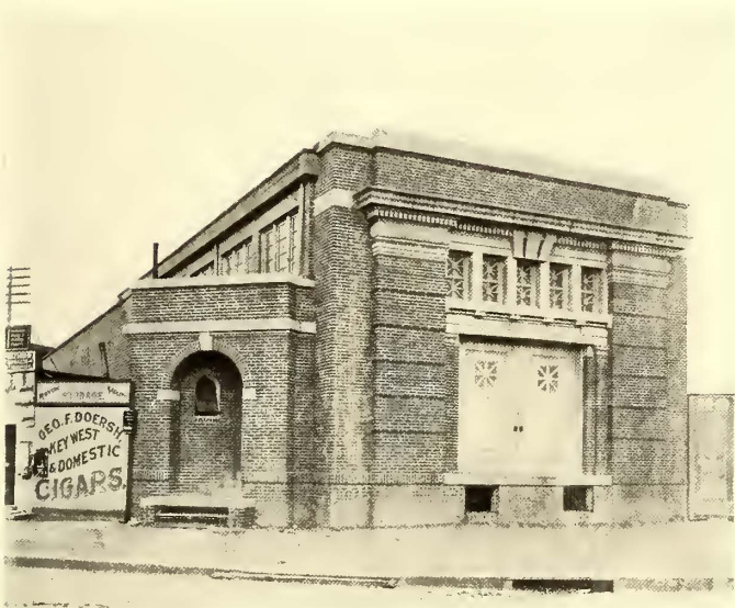
EXTERIOR SUB-STATION AT FIFTY-SECOND STREET AND LANCASTER AVENUE
