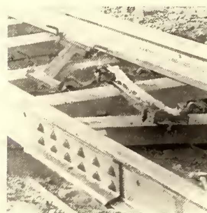
Joint with Moulds Removed
