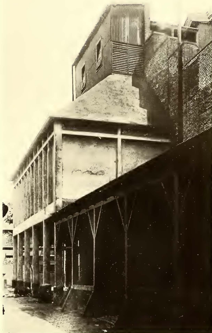
CONCRETE CINDER BIN AT THIRTEENTH AND MT. VERNON STREETS POWER HOUSE
