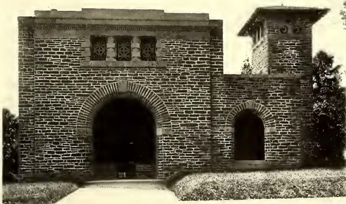
EXTERIOR GLENSIDE SUB-STATION
