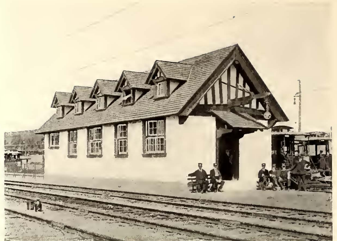
BUILDING FOR CONDUCTORS AND MOTORMEN AT WILLOW GROVE TERMINAL
