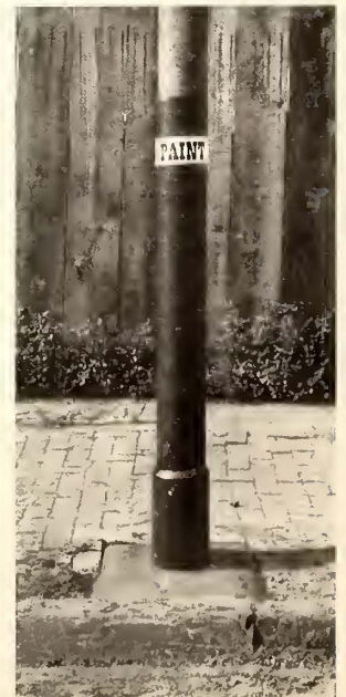
Finished Pole, with Sleeve and Concrete in Place
