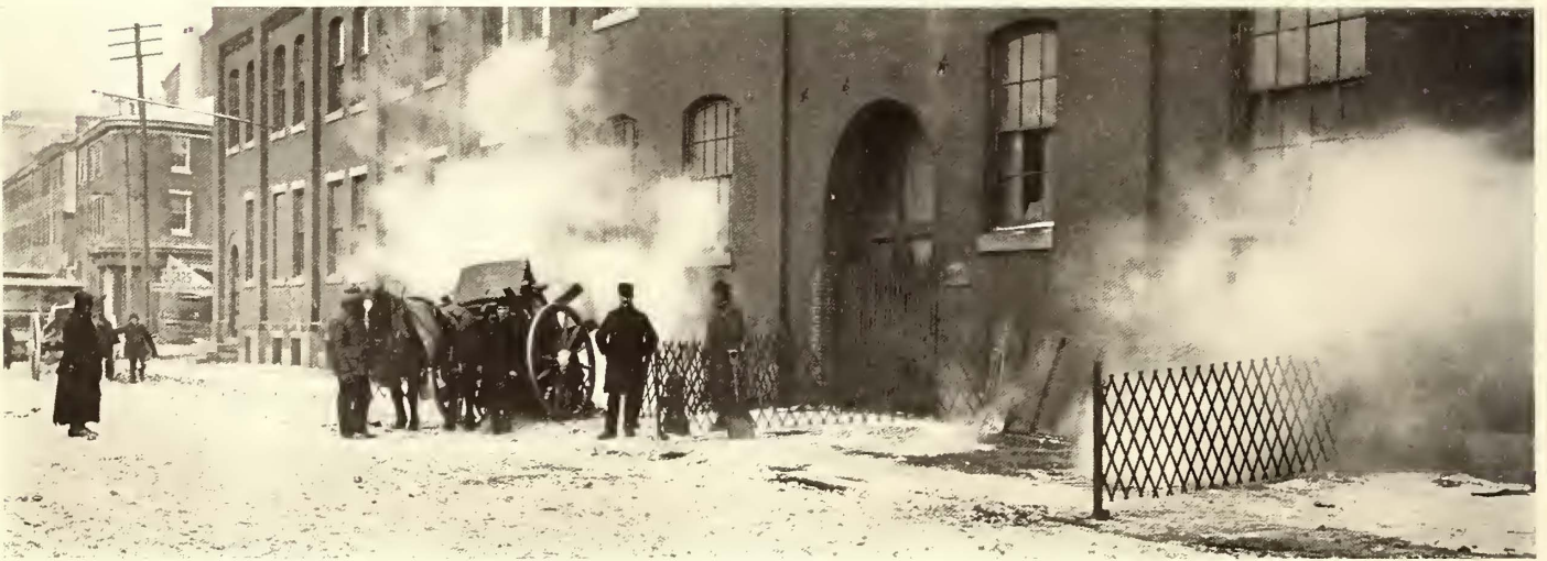
DUMPING SNOW INTO MELTING PITS
