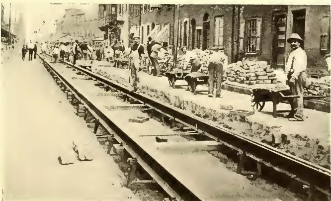
TRACK READY FOR CONCRETE
