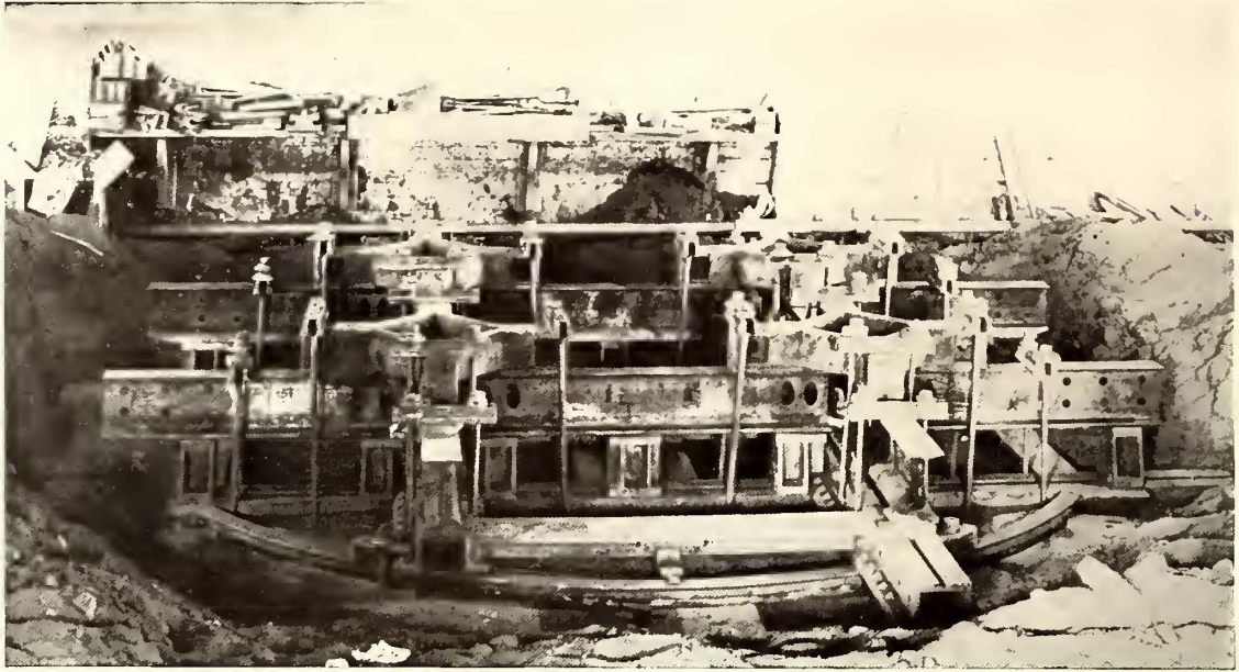
UNIVERSAL CLAMP FOR ASSEMBLING CROSSINGS
