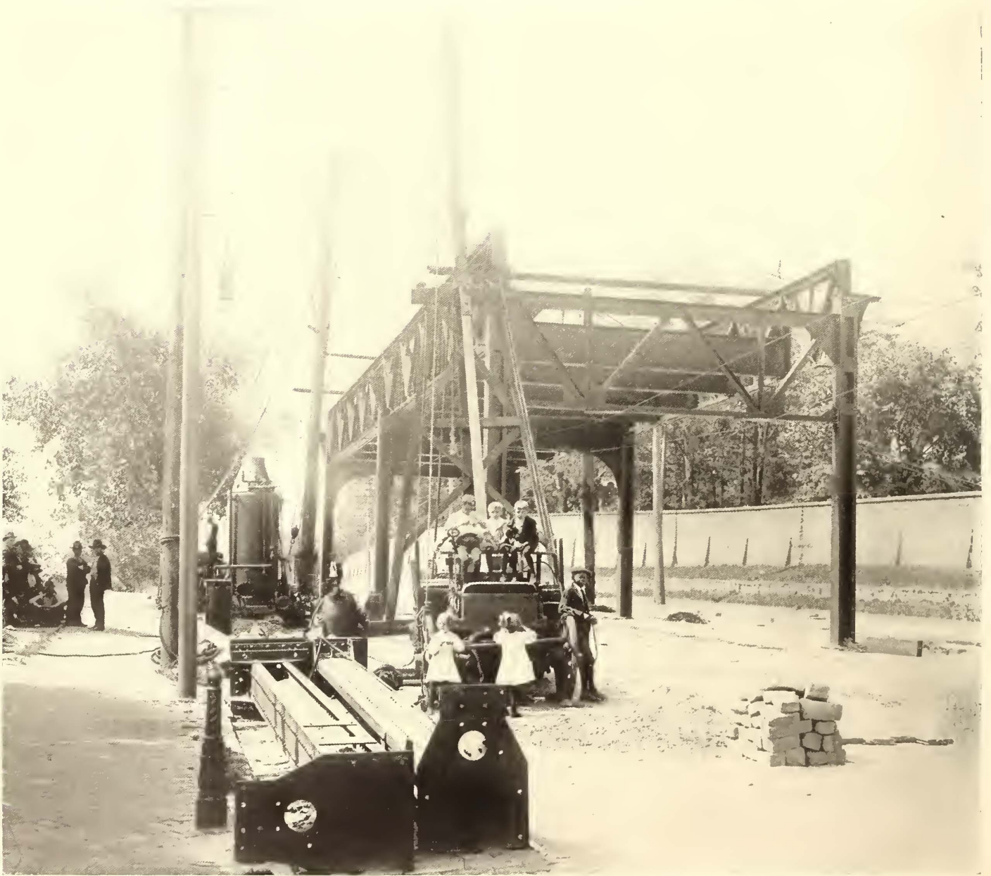
VIEW TAKEN EARLY IN SEPTEMBER OF THIS YEAR, SHOWING FIRST SECTION OF ELEVATED STRUCTURE ON WEST MARKET STREET
