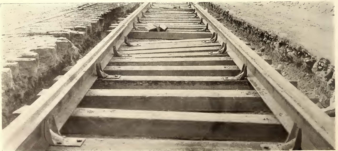
TRACK WITH CHAIR BRACE CONSTRUCTION
