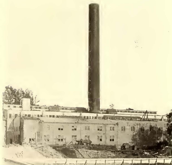
EXTERIOR OF GENERATING STATION AT SECOND STREET AND WYOMING AVENUE
