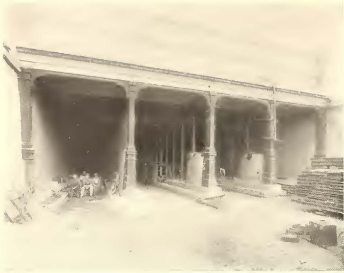
VIEW OF WEST PORTAL TO SUBWAY
