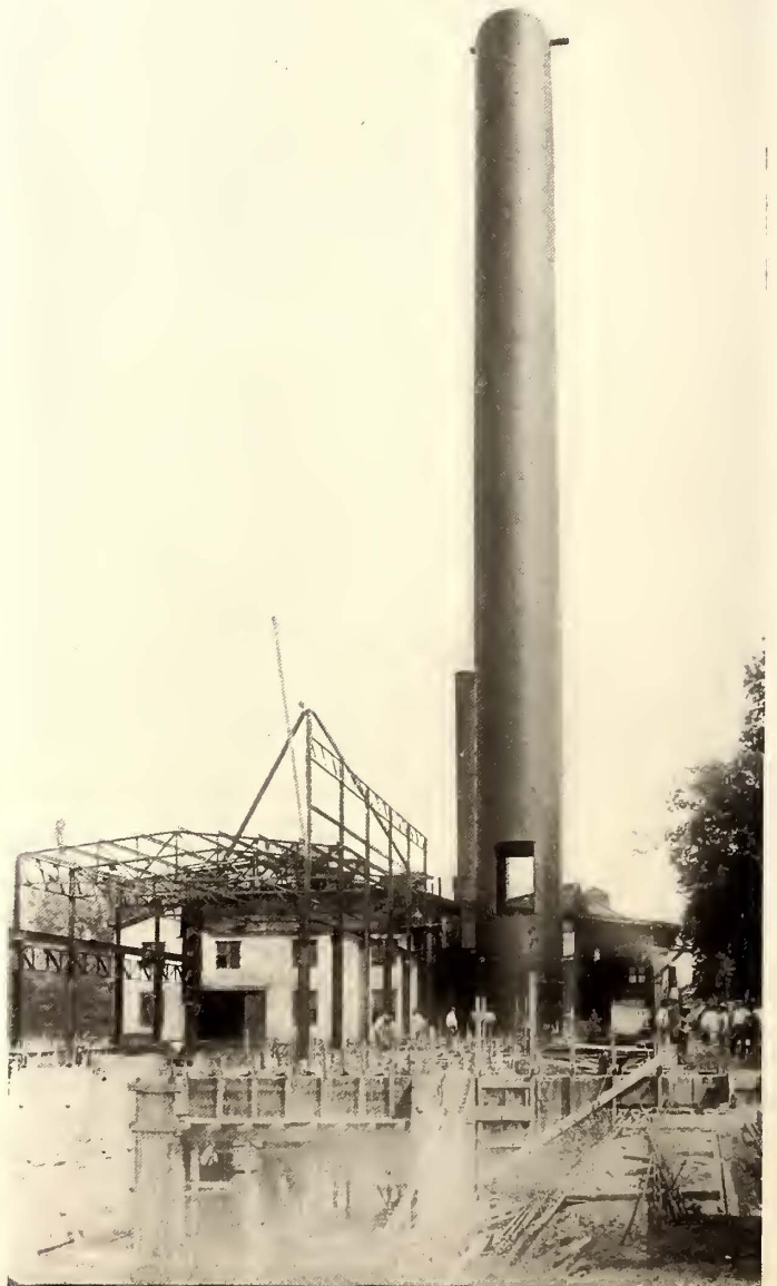
EXTERIOR GENERATING STATION AT SECOND STREET AND WYOMING AVENUE DURING CONSTRUCTION
