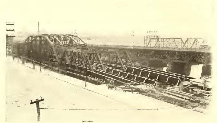
SCHUYLKILL RIVER BRIDGE, LOOKING WEST, SHOWING ELEVATED TRACKS ON INCLINE IN CENTER, AND SURFACE TRACKS AT SIDES
