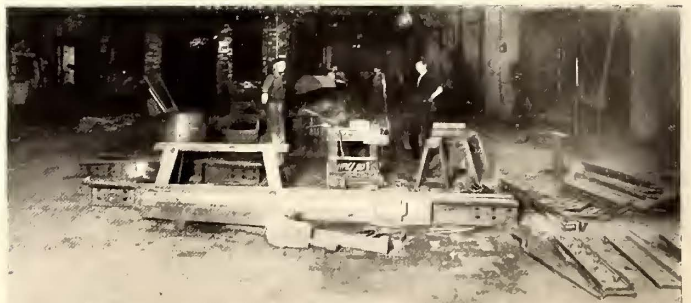
BLACKSMITH SHOP, ROADWAY SHOPS
