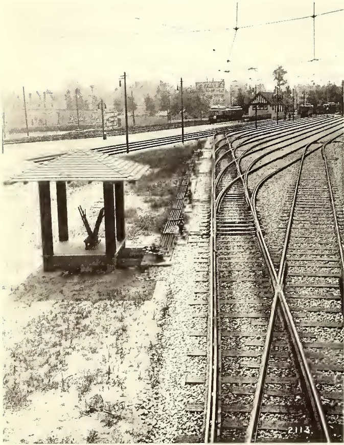
HARDENED STEEL SWITCHES AT ENTRANCE TO WILLOW GROVE TERMINAL
