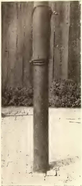
Pole Before Digging—Sleeve is Held Temporarily by Rope
