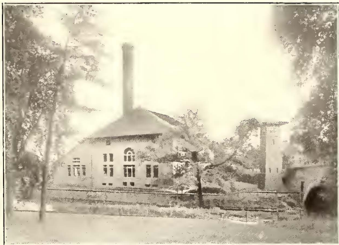
EXTERIOR OGONTZ POWER HOUSE
