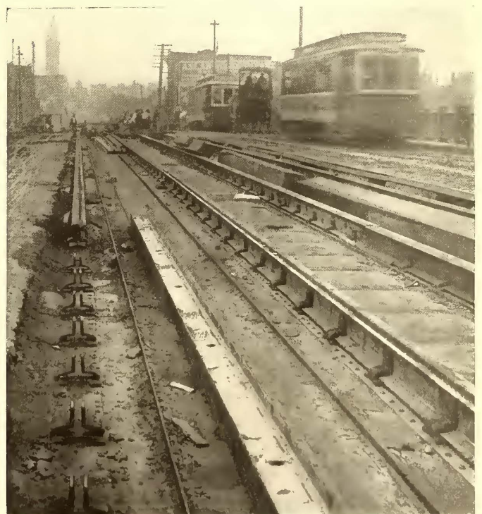
DETAILS OF SPECIAL RAIL CHAIRS ON BRIDGES
