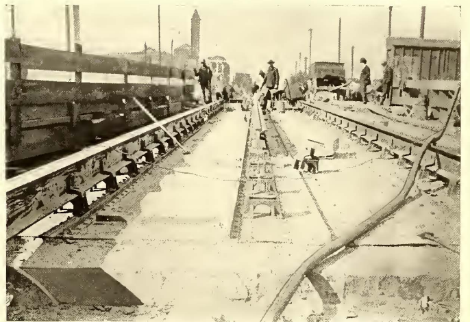
SPECIAL RAIL CHAIRS USED ON BRIDGE WORK
