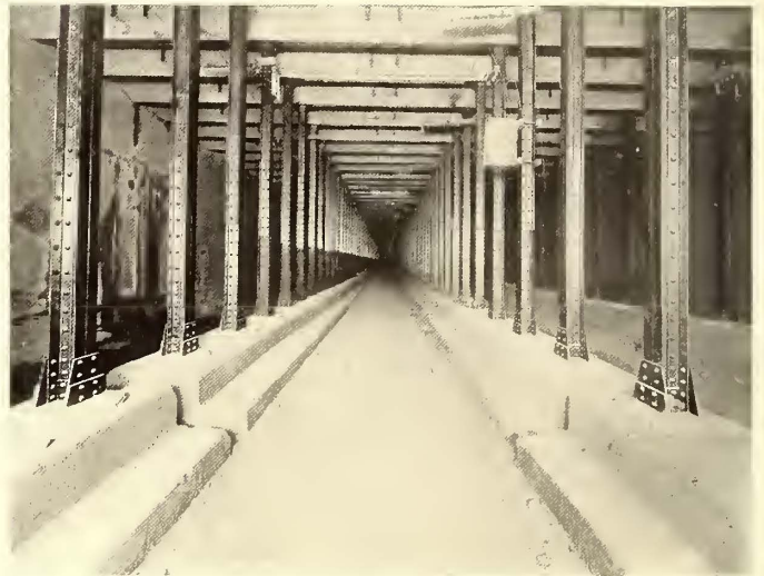
TYPICAL VIEW IN SUBWAY BEFORE TRACKS WERE LAID
