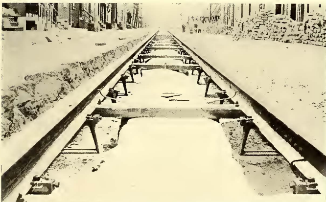
TRACK WITH YOKES ATTACHED PRIOR TO PLACING CONCRETE
