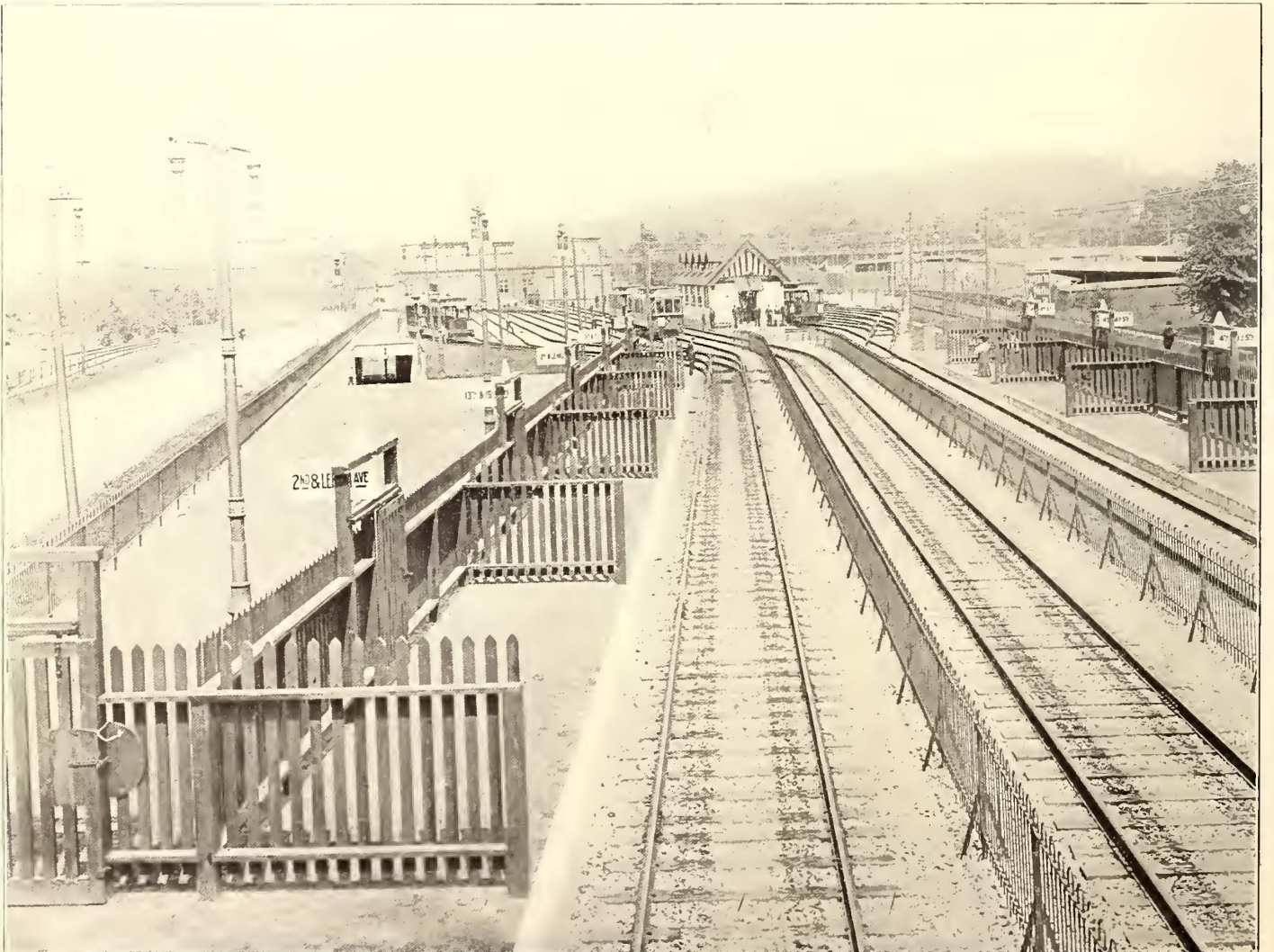
WILLOW GROVE TERMINAL, SHOWING GATES AND INDICATING SIGNS ON LOADING PLATFORMS
