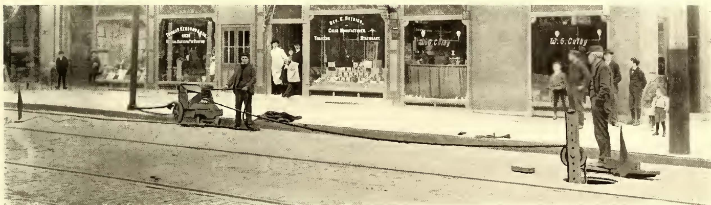
ELECTRIC WINCH DRAWING CABLE THROUGH DUCTS
