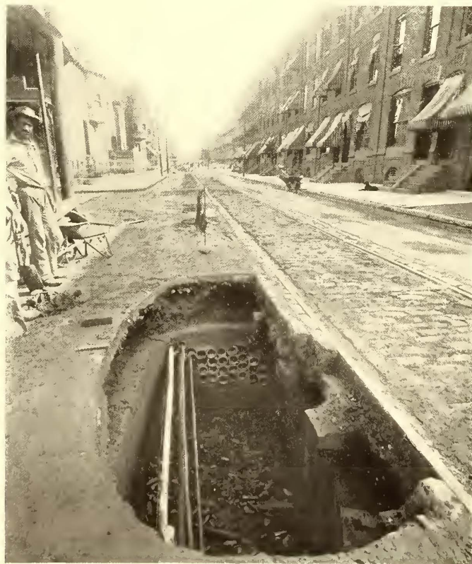
CABLES AND DUCTS IN CABLE CONDUIT
