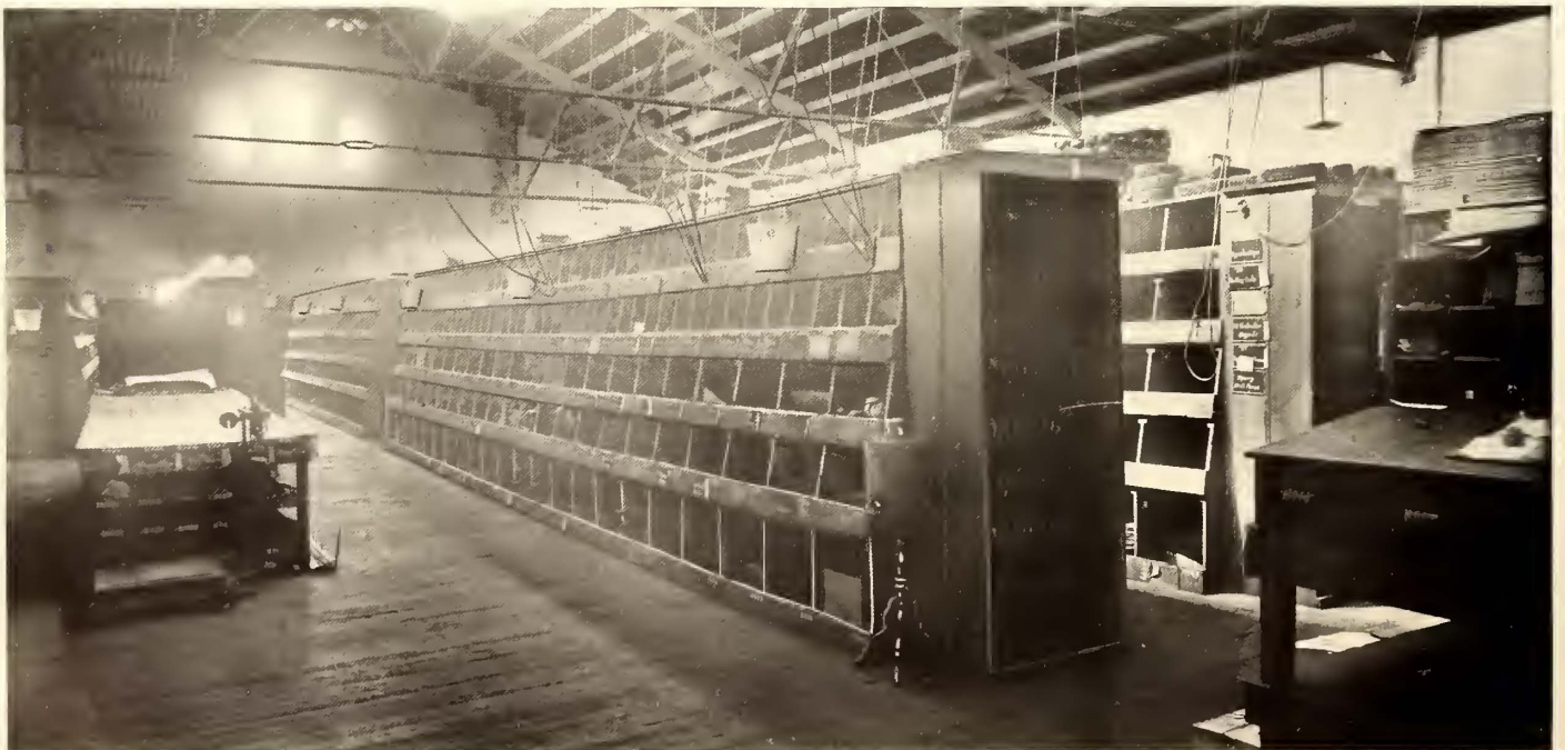
GENERAL STOREROOM, EIGHTH AND DAUPHIN STREETS
