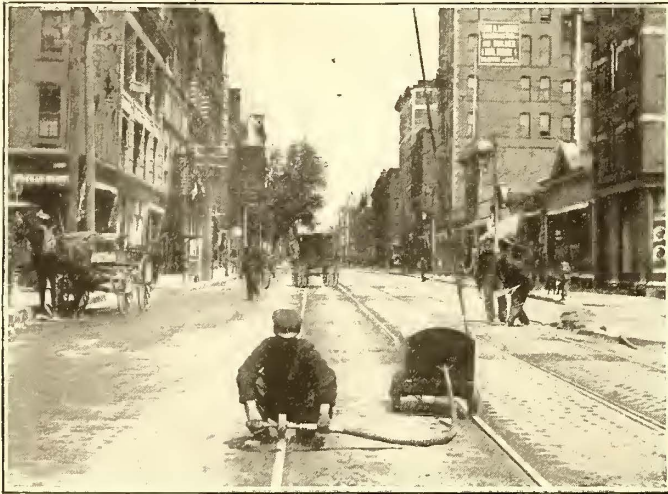
GRINDER FOR SMOOTHING JOINT
