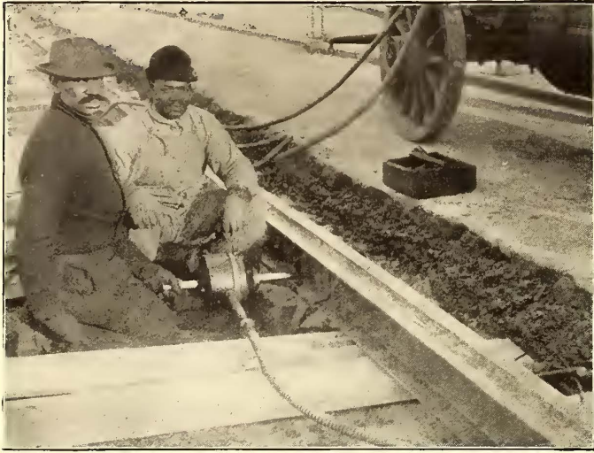
FIG. 5.—REAMING HOLES
