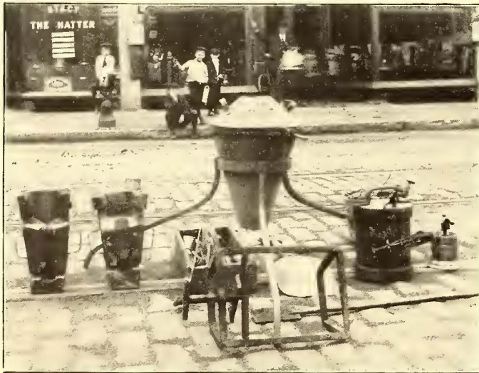
COMPLETE WELDING OUTFIT FOR THE THERMIT RAIL-WELDING PROCESS
