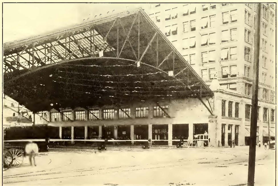
FIG. 4.—ENTRANCE GATES TO PASSENGER TRAIN SHED
