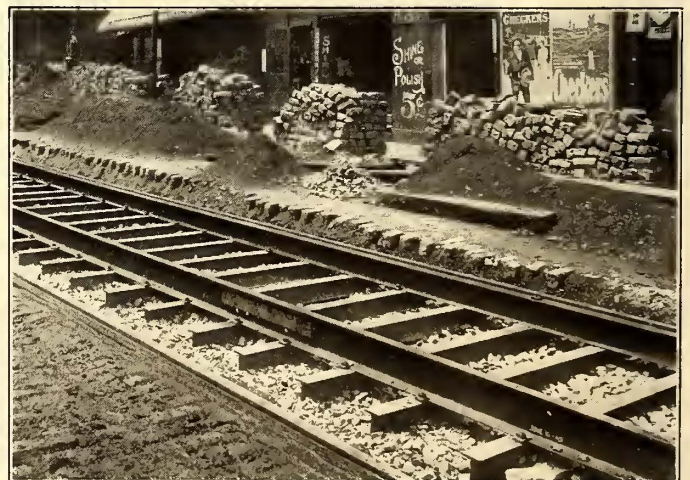
NEW TRACK CONSTRUCTION WITH STEEL TIES
