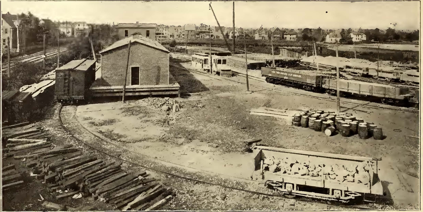
STOCK YARDS OF THE CLEVELAND ELECTRIC RAILWAY
