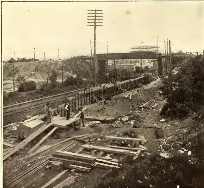
HOLDING THE RETAINING WALL
