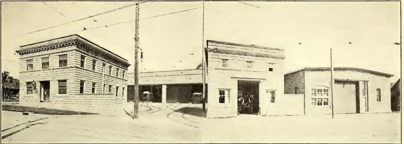
TOPEKA RAILWAY BUILDINGS, FROM STREET
