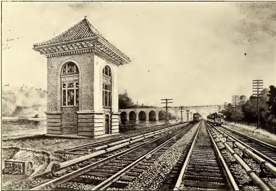
APPEARANCE OF A CABLE TOWER AND PART OF THE TRANSMISSION AND THIRD-RAIL SYSTEM ON THE LINE OF THE NEW YORK CENTRAL & HUDSON RIVER RAILROAD
