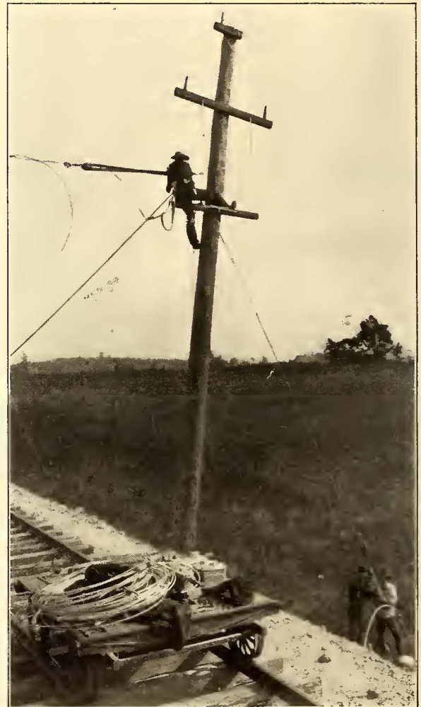
FASTENING GUY ANCHORS AND PULLING UP SPAN WIRE
