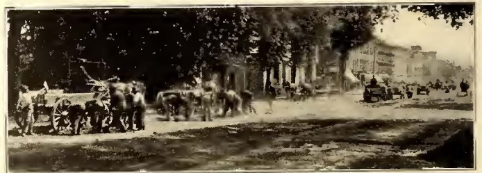
EXCAVATING ON MAIN STREET, PALMYRA, N. Y.
