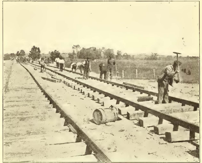
TRACK GANG SPIKING DOWN RAILS ON SECOND TRACK
