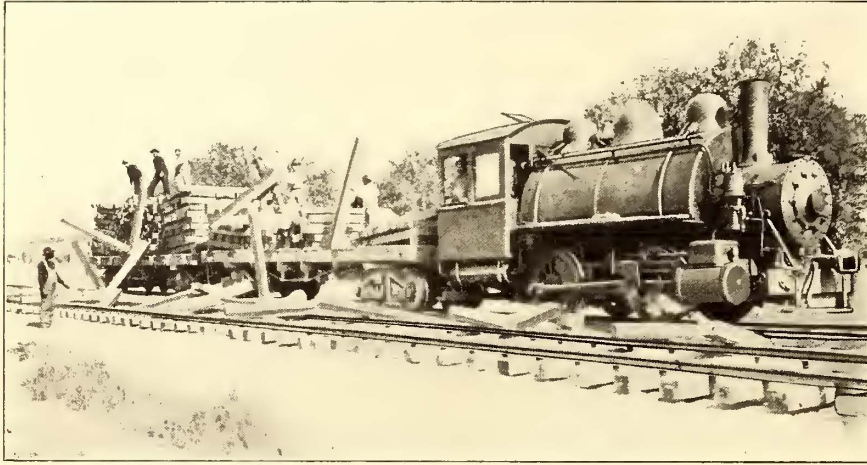
UNLOADING TIES FROM CONSTRUCTION TRAIN
