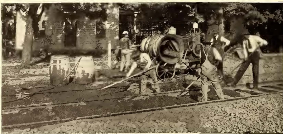
GASOLINE ENGINE-DRIVEN PORTABLE MIXER USED IN WORK IN VILLAGE STREETS
