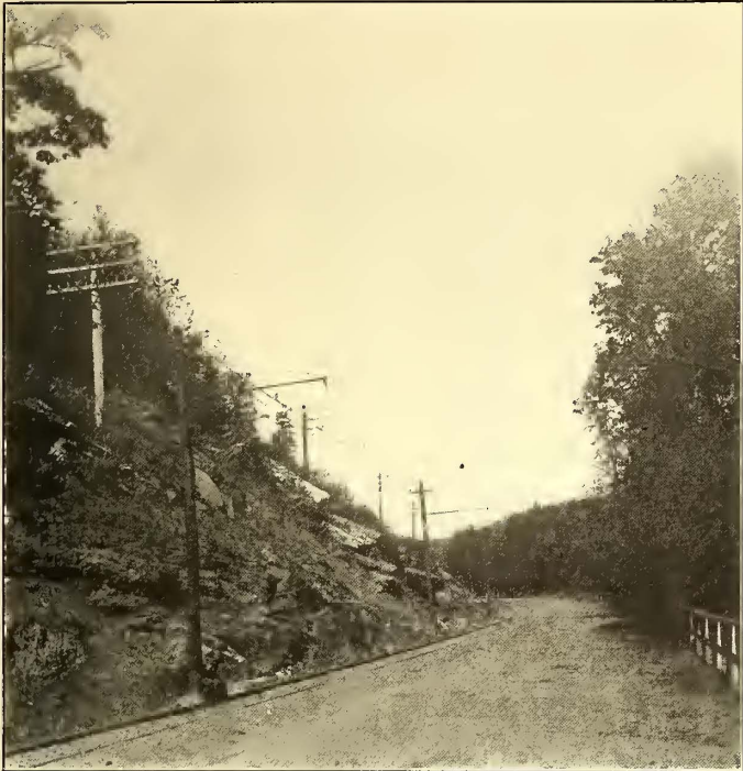
VIEW OF A PART OF THE PUBLIC HIGHWAY WHICH WAS WIDENED BY BLASTING THE ROCK ALONGSIDE
