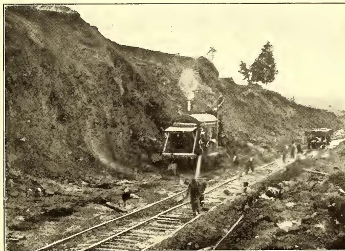
EXCAVATING IN 54,000-CU. YD. CUT NEAR PALMYRA
