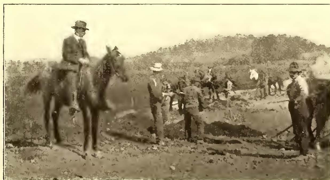
GRADING WITH TEAMS. THE TIMEKEEPERS ARE MOUNTED ON HORSEBACK
