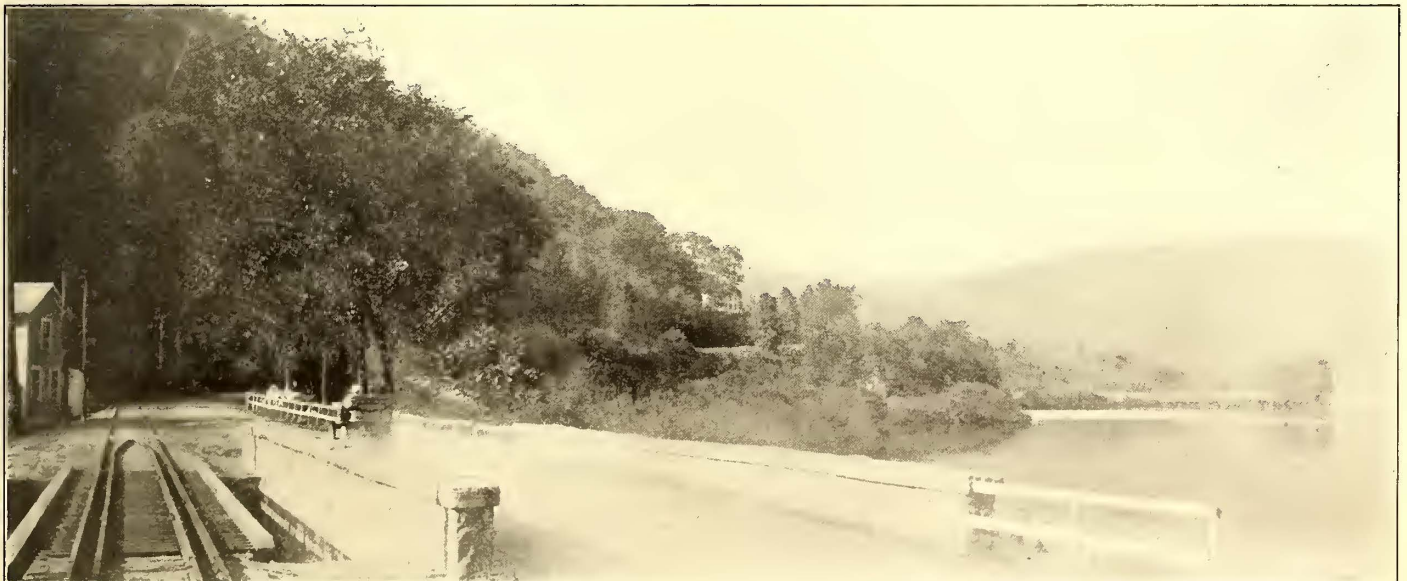
ROAD AND RAILWAY BRIDGES ACROSS THE WESTFIELD RIVER, ON THE LINE OF THE WESTERN MASSACHUSETTS RAILWAY, BETWEEN WORONOCO PARK AND HUNTINGTON
