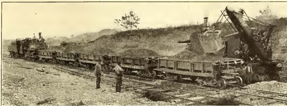
METHOD OF LOADING AND HAULING GRAVEL FOR BALLAST
