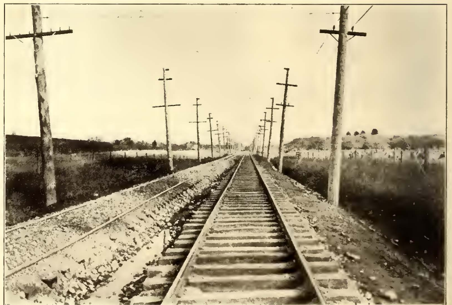
ONE TRACK GIVEN FIRST LIFT, OTHER UNBALLASTED
