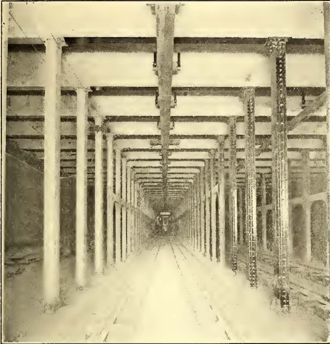
LOOKING UP AN EXPRESS TRACK. A THIRD RAIL WILL BE USED LATER INSTEAD OF THE OVERHEAD WIRE SHOWN
