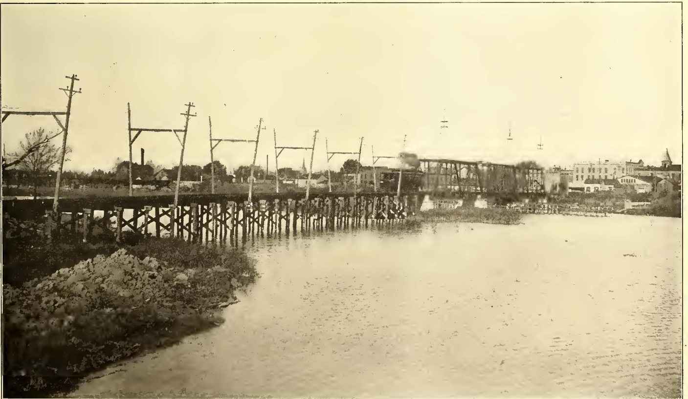
VIEW OF SWING BRIDGE AND TRESTLE AT OAK HARBOR, SHOWING ALSO THE HIGH-TENSION TOWERS CROSSING THE STREAM
