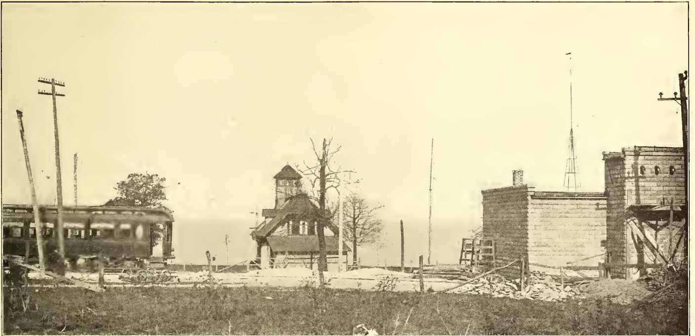
CAR LEAVING THE MARBLEHEAD TERMINUS OF THE TOLEDO, PORT CLINTON & LAKESIDE RAILWAY. THE CONCRETE SUBSTATION AT THIS TERMINAL IS SHOWN AT THE RIGHT
