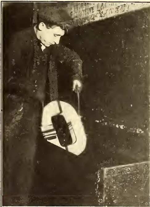
DIPPING FIELD COILS, MONTREAL STREET RAILWAY SHOPS
