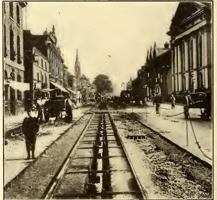
COMPLETED CONDUIT BEFORE FILLING WITH CONCRETE
