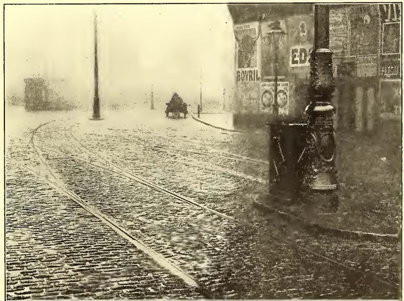
FIG. 3.—VIEW AT A JUNCTION, SHOWING AN INSTALLATION OF AN AUTOMATIC TRACK SWITCH. THE SWITCHING MECHANISM IS IN THE BOX NEXT TO THE POLE ON THE RIGHT
