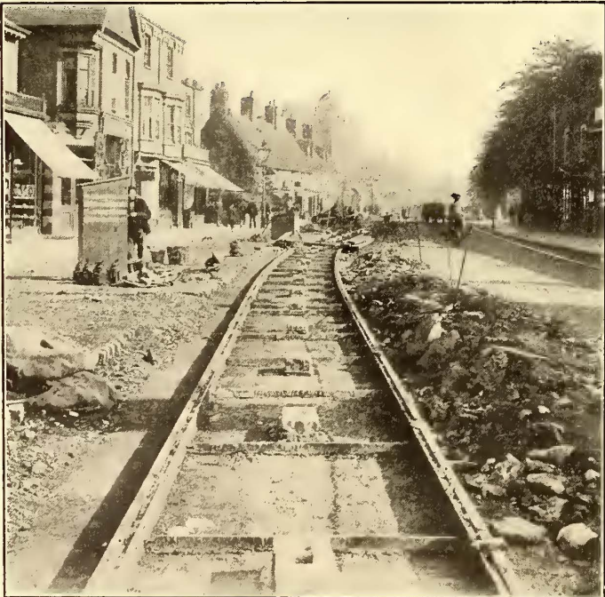
CONDITION OF TRACK WHEN PAVING
