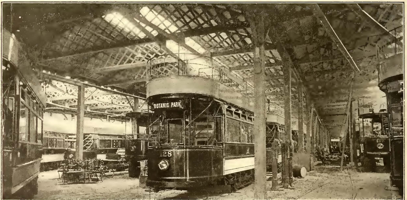
INTERIOR VIEW OF THE BELFAST TRAMWAYS CAR HOUSE AT FALLS ROAD
