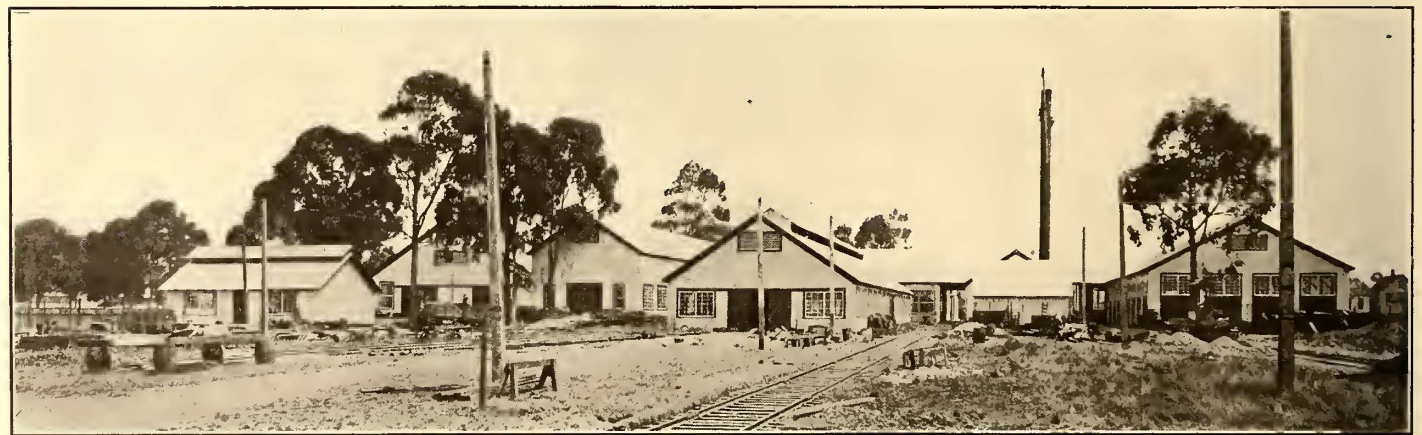
GENERAL VIEW, OAKLAND TRACTION SHOPS
