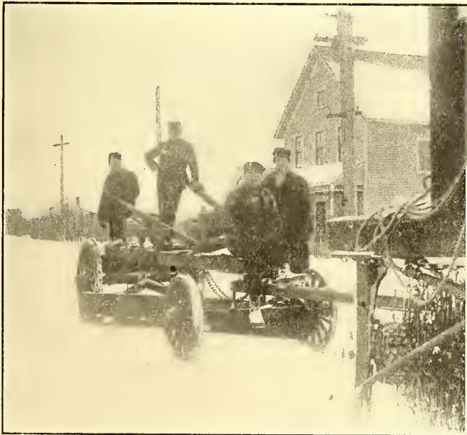
SCRAPER USED FOR CUTTING DOWN RIDGE BETWEEN RAILS
