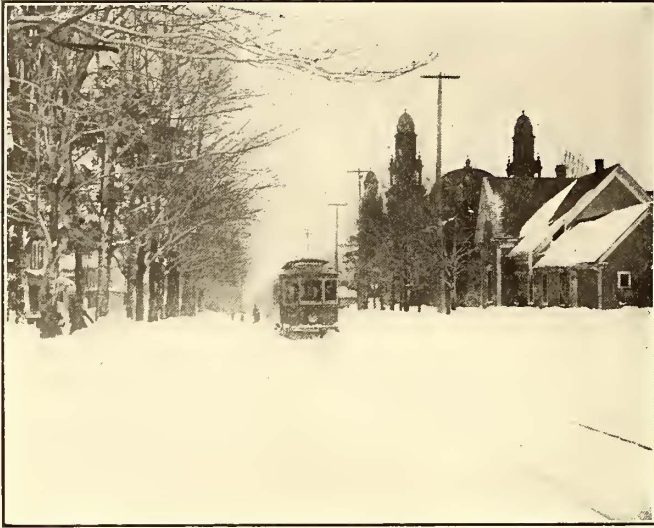
TYPICAL STREET SCENE IN MARQUETTE DURING WINTER
