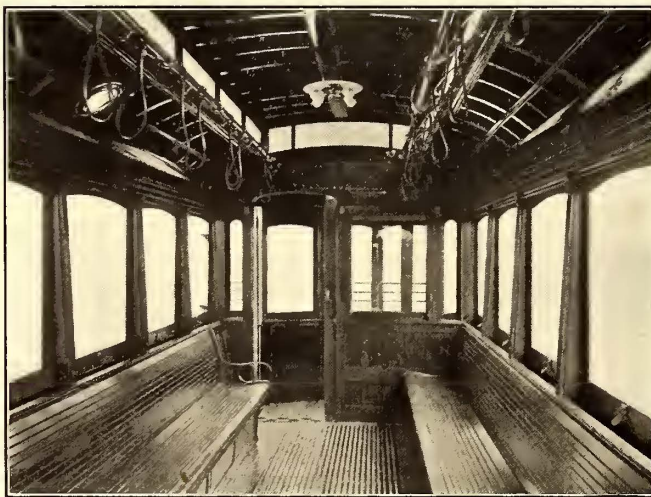
LONGITUDINAL SEATING AND SEMI-ACCELERATOR DOOR OF VINCENNES CAR
