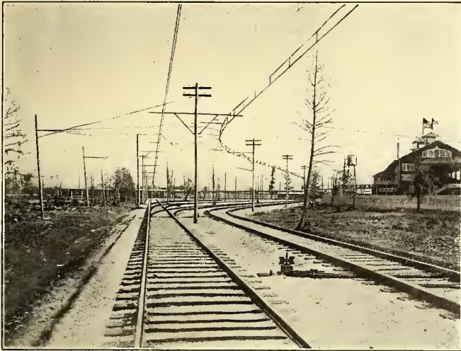
DIRECT-CURRENT CATENARY AT NEW ORLEANS
