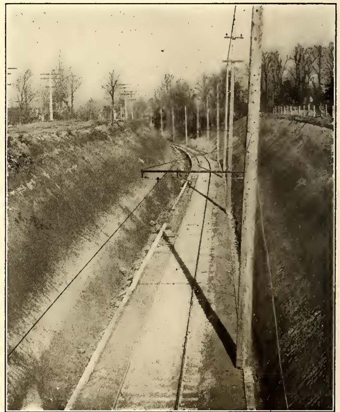
CUT ON SULLIVAN LINE, WITH CONCRETE PROTECTION
