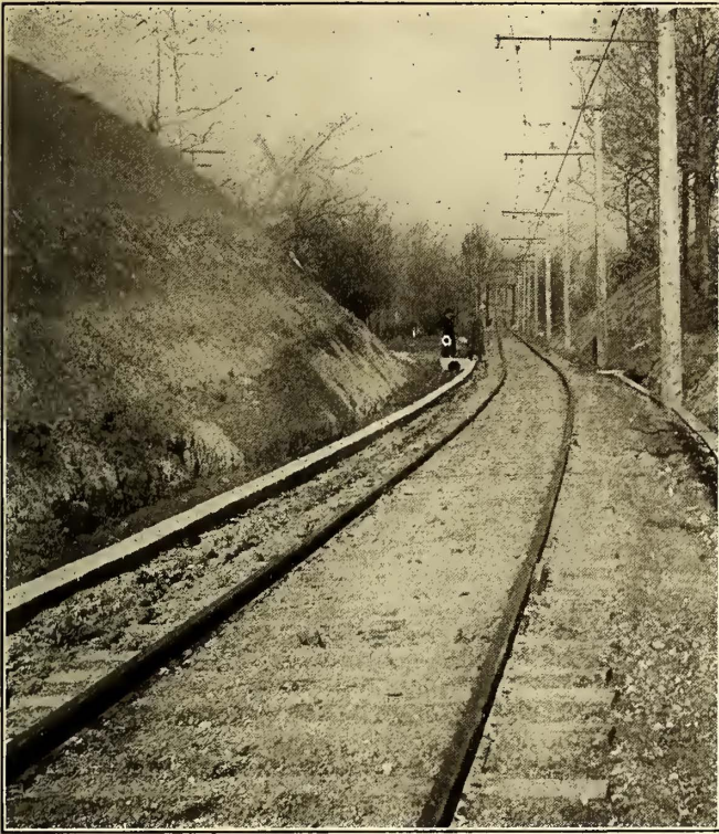
CUT ON SULLIVAN LINE, SHOWING CONCRETE WORK TO PROTECT GRADES FROM WASHING
