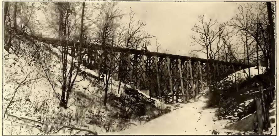
TRESTLE BRIDGE ON ST. MARY'S LINE
