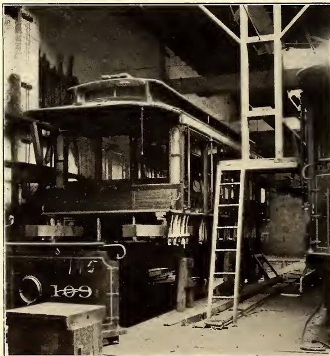
FIG. 5.—ELEVATED PLATFORMS IN CARPENTER SHOP, ST. JOSEPH, MO.
