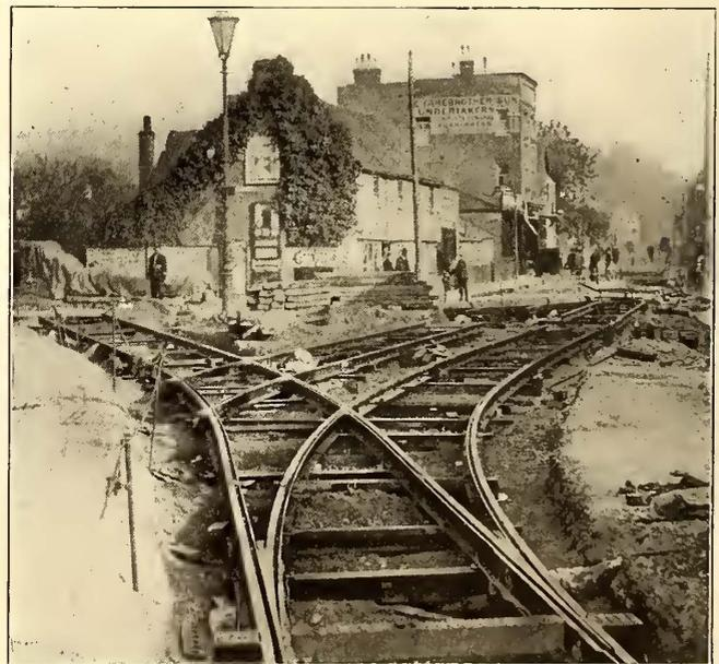
JUNCTION OF KINGSTON ROAD AND LONDON ROAD. SHOWING METHOD OF LAYING STEEL TIES
