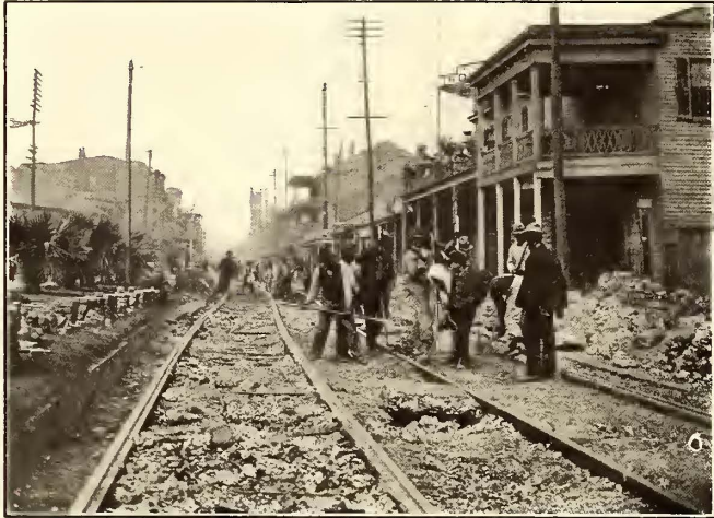
TEARING OUT OLD TRACK WORK IN ASPHALT STREET, NEW ORLEANS
