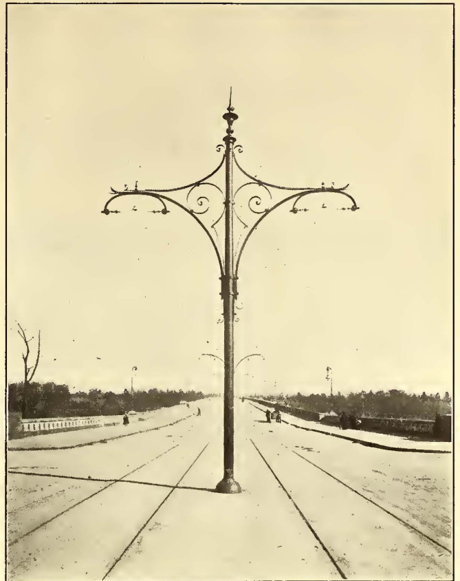
ARTISTIC OVERHEAD CONSTRUCTION ON WASHINGTON BRIDGE
