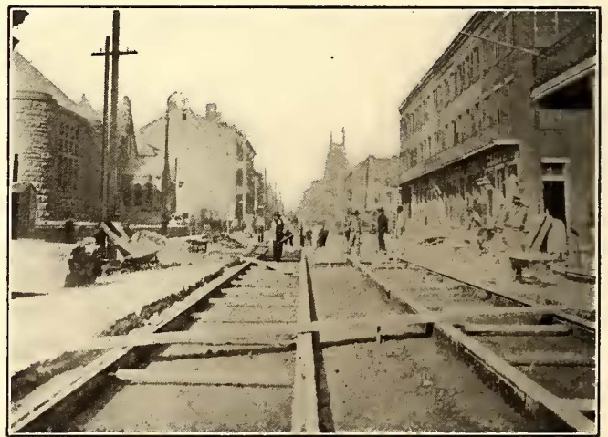
CONCRETED TRACK READY FOR PAVING, NEW ORLEANS
