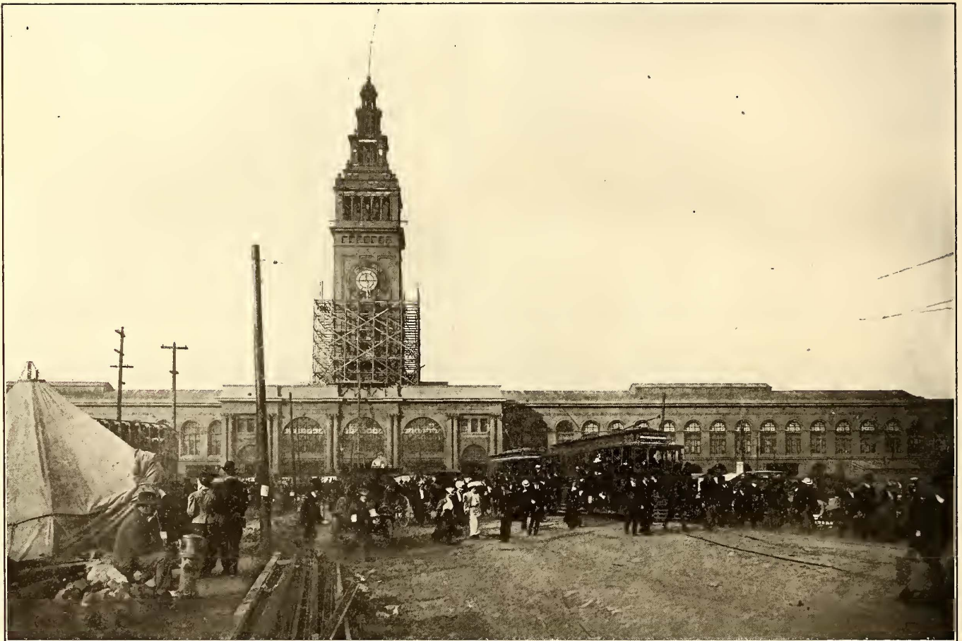
VIEW REPRODUCED FROM PHOTOGRAPH TAKEN MAY 6, 1906, INDICATING RESTORATION OF ELECTRIC RAILWAY SERVICE TO SAN FRANCISCO'S FAMOUS FERRY BUILDING
