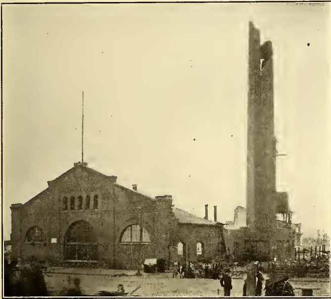
RUINS OF THE VALENCIA & MARKET STREETS CABLE POWER HOUSE, OFFICES AND MAIN REPAIR SHOPS OF THE UNITED RAILROADS, OF SAN FRANCISCO. THE BRICK-RIBBED CHIMNEY WAS CRACKED TO THE FOUNDATIONS BY THE EARTHQUAKE
