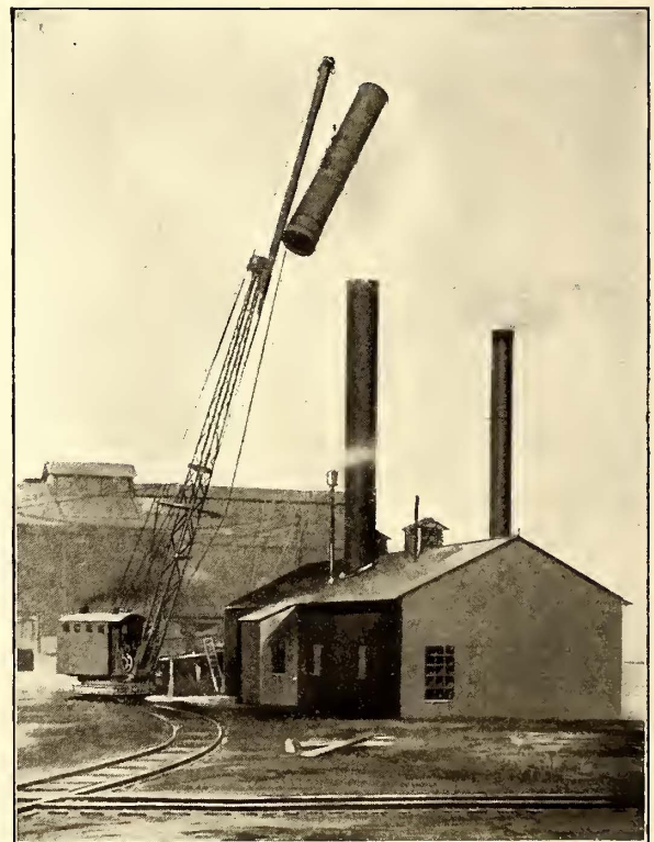
LOCOMOTIVE CRANE USED FOR ERECTING A SMOKESTACK
