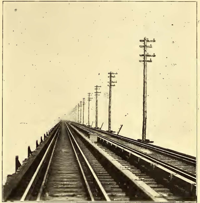
FIG. 13.—WOODEN-POLE CONSTRUCTION ON JAMAICA BAY TRESTLE
