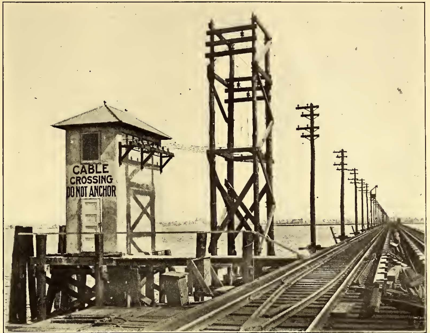
FIG. 8.—ARRESTER HOUSE AT BROAD CHANNEL DRAWBRIDGE
