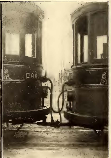
FIG. 5.—COUPLING BETWEEN TWO CARS
